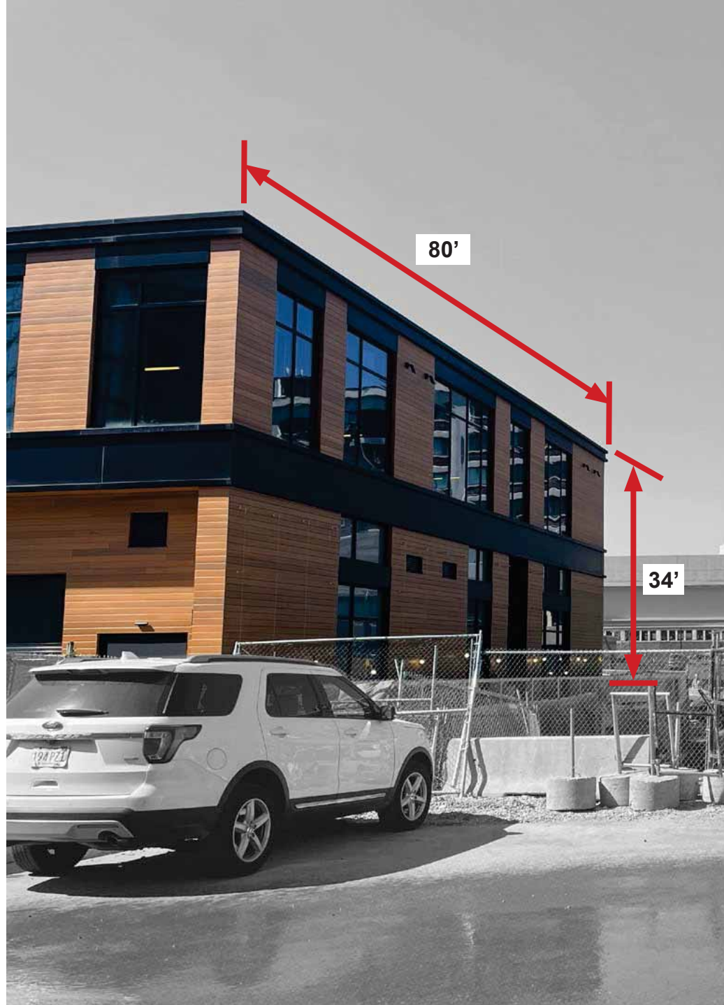
Parcel Q1 - West Facade
