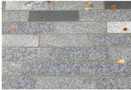
Stone Setts Pavement
