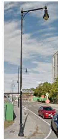
Light Pole - Street
