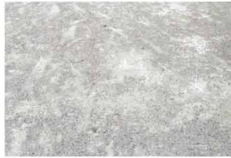
Decomposed Granite Pavement
