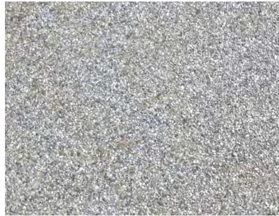
Exposed Aggregate Concrete Pavement
