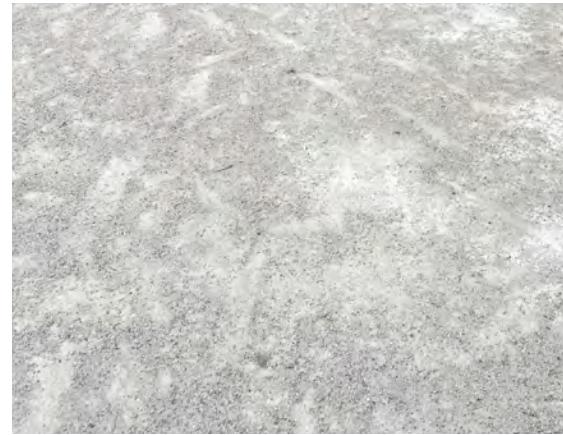
Decomposed Granite Pavement
