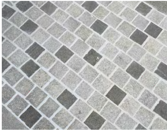
Stone Setts Pavement
