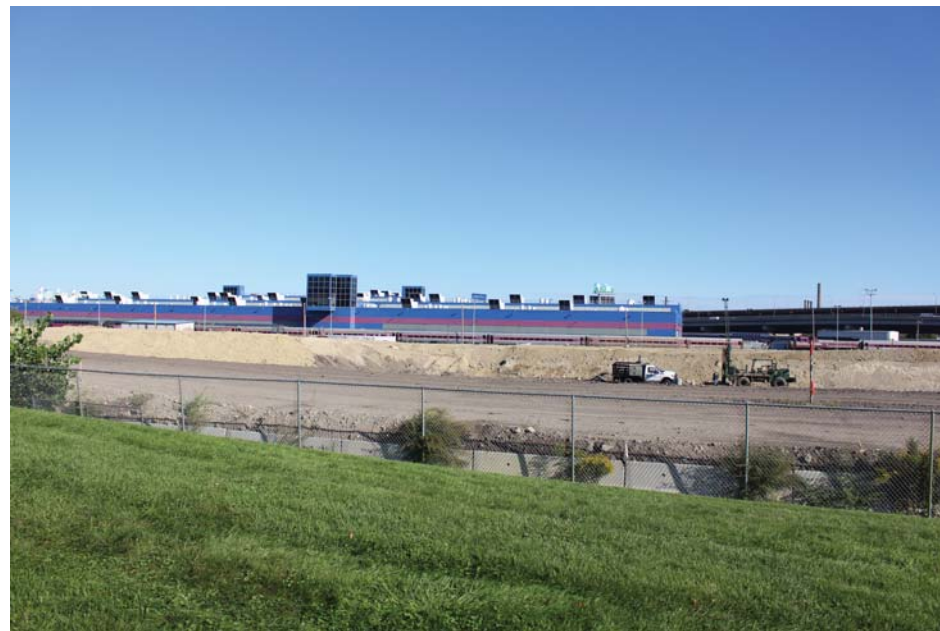
5- VIEW FROM NORTHPOINT COMMON LOOKING AT PARCEL JK
