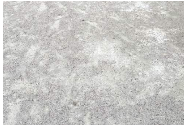
Decomposed Granite Pavement
