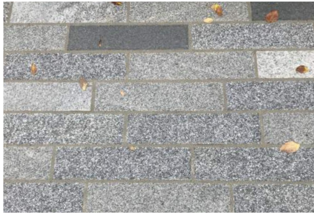
Stone Setts Pavement
