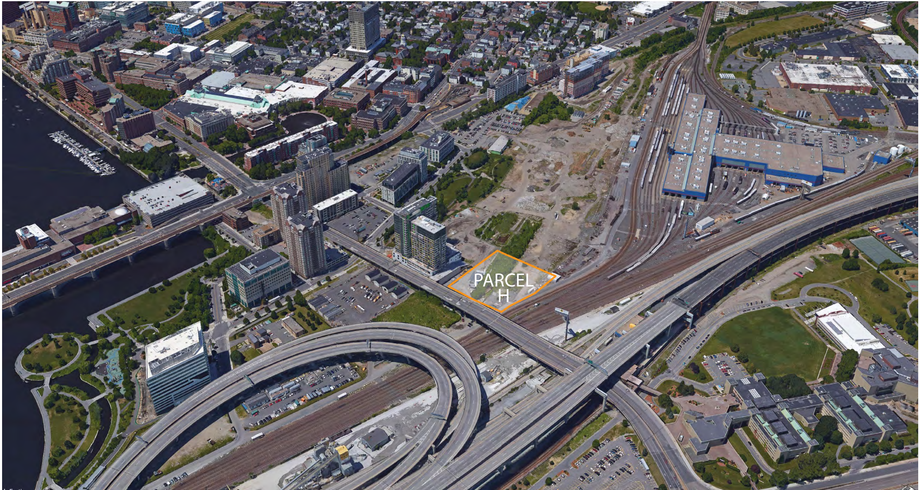
EXISTING AERIAL PHOTO: NORTHEAST
