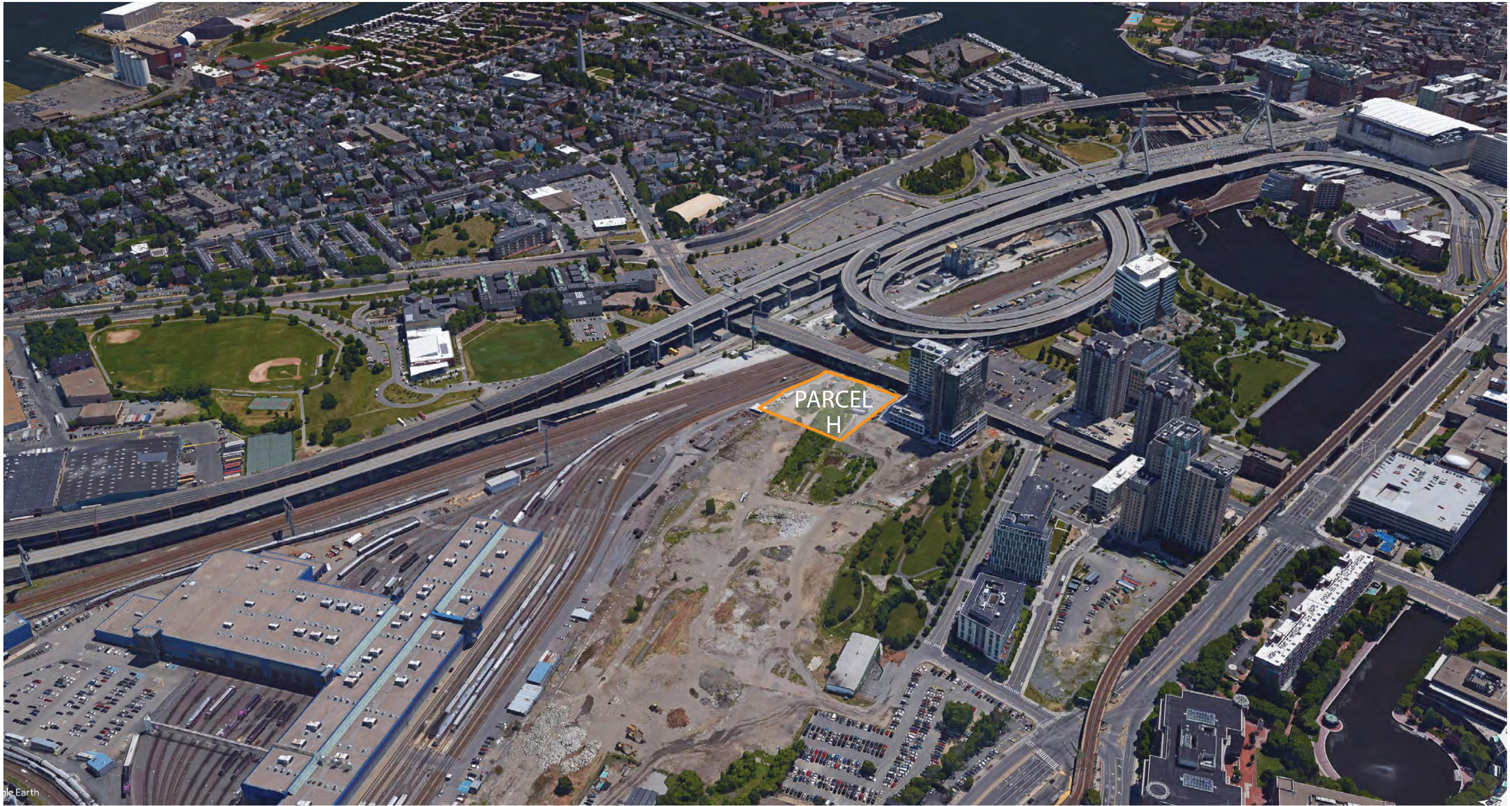
EXISTING AERIAL PHOTO: SOUTHWEST
