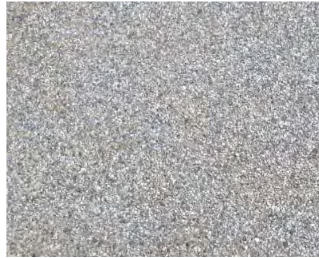
Exposed Aggregate Concrete Pavement
