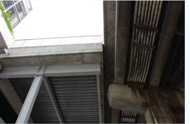
Gilmore Bridge, Existing Condition
