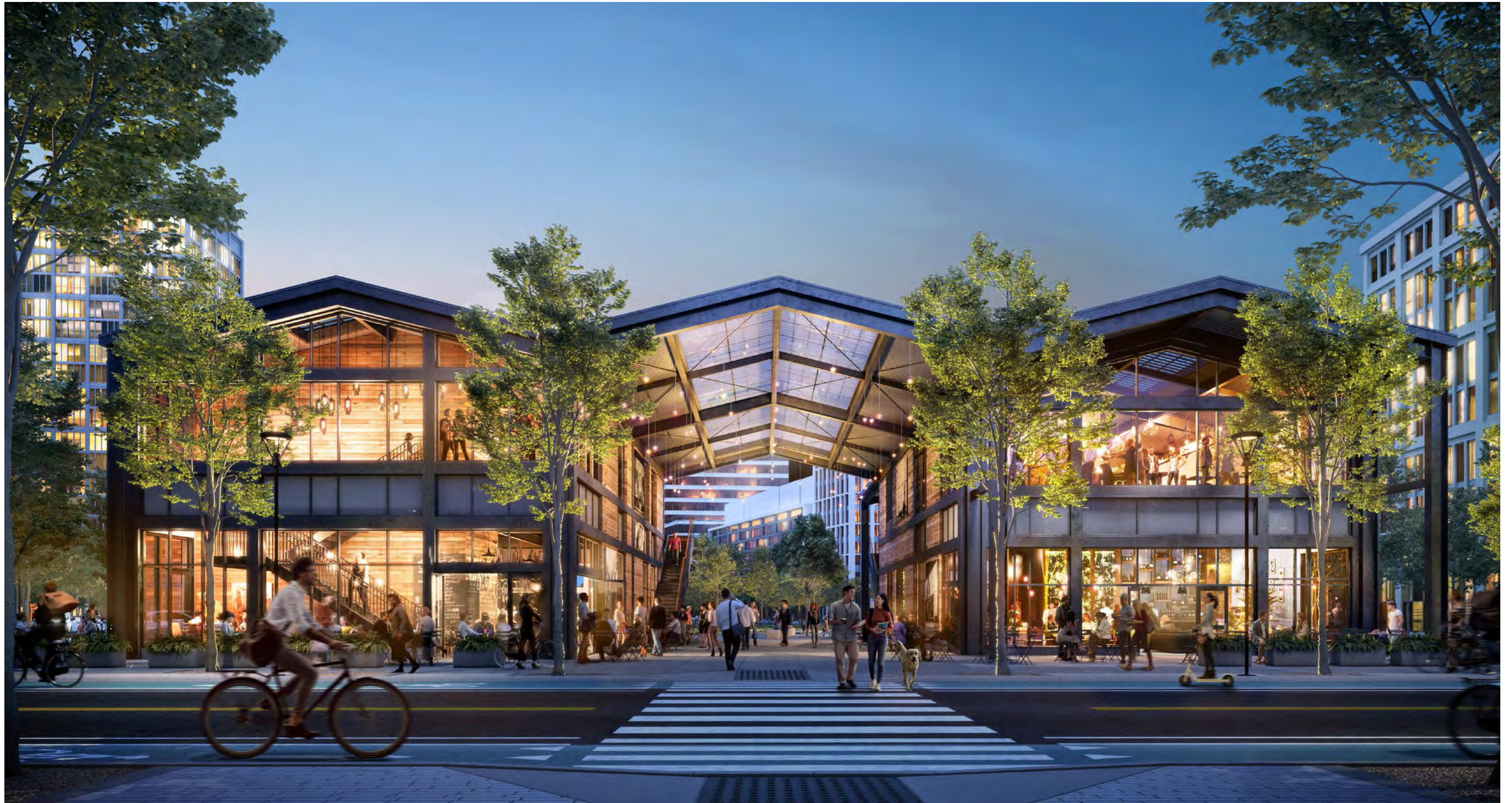
VIEW LOOKING EAST ACROSS NORTH FIRST STREET THROUGH OPEN CENTER BAY TOWARDS COMMON
