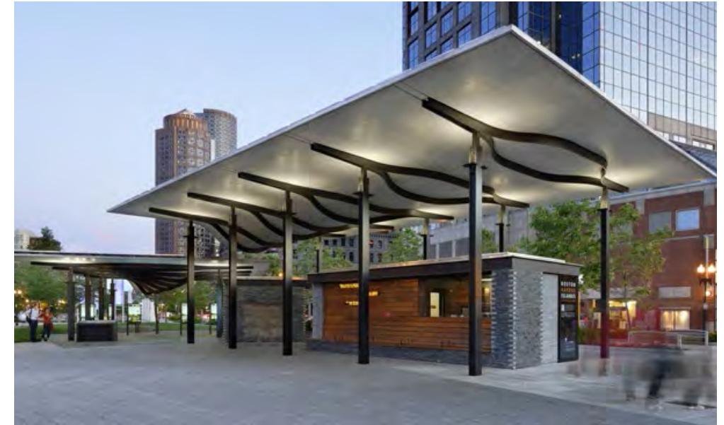
Pavilions in a park and plaza: Boston Harbor Islands Pavilion
