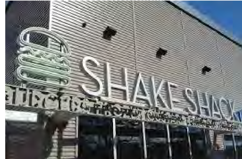
Preferred: Internally illuminated individual translucent letters with opaque sides. Lighting to be mounted inside each individual letter. See Zoning Article 7 for additional requirements.
