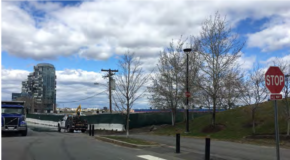
3 - View from Northpoint Boulevard looking west
