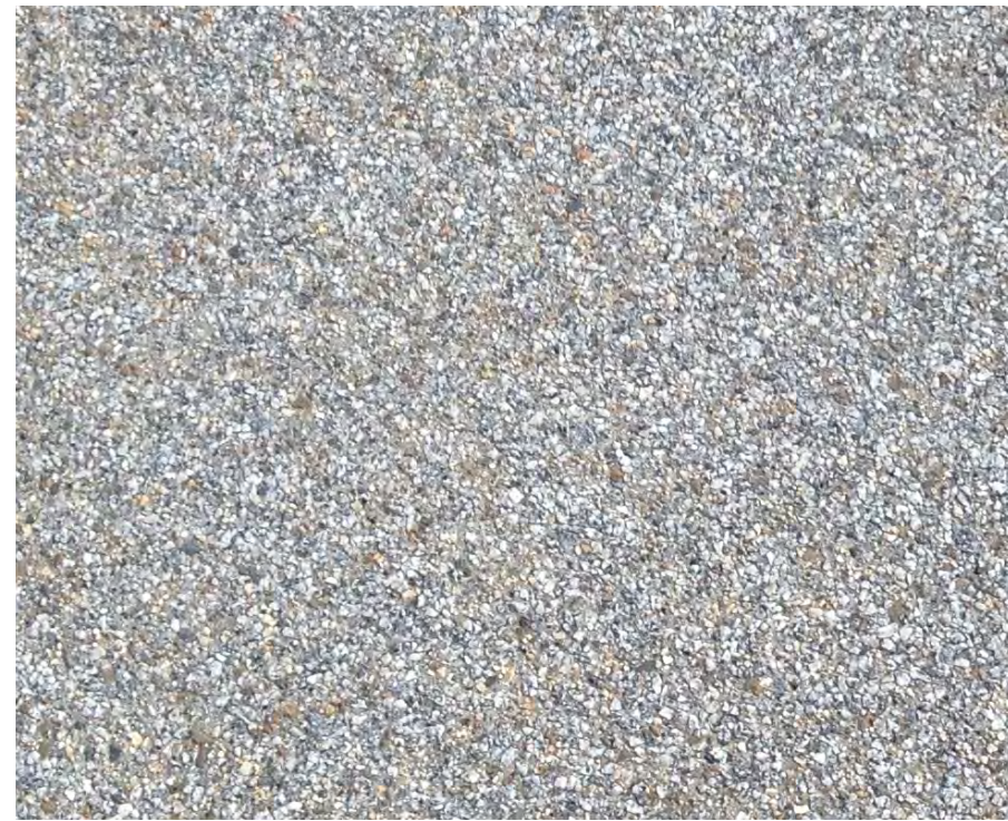
Exposed Aggregate Concrete Pavement
