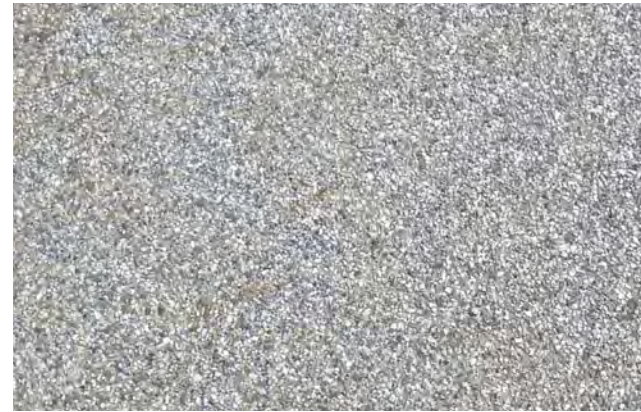
Exposed Aggregate Concrete Pavement
