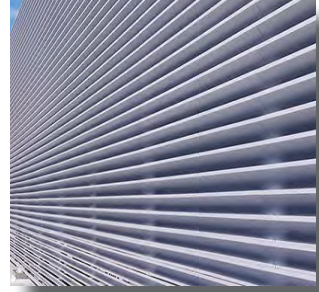
LOUVER WALL MECHANICAL SCREEN
