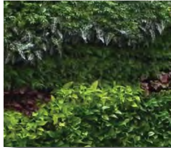
LIVING WALL GROWTH WALL ON SOUTH FACADE
