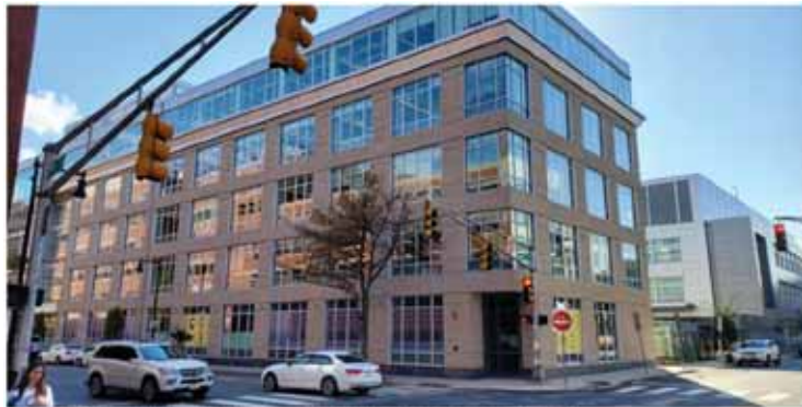
VIEW FROM FIRST STREET @ CHARLES STREET CORNER
