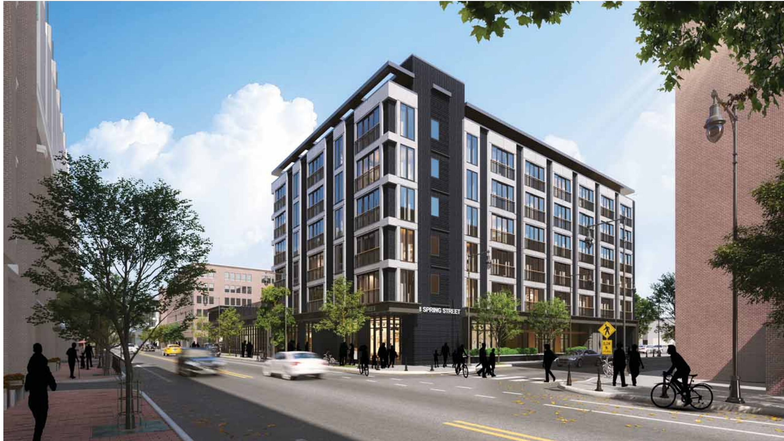
VIEW FROM FIRST ST. AND SPRING ST.
