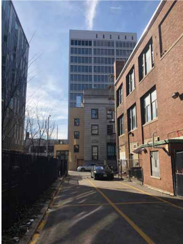
View from Back Alley Looking at Temple Street
