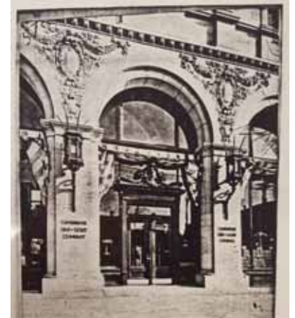
Closeup View of Facade from Massachusetts Ave
