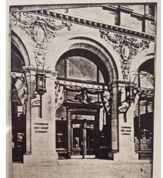
Closeup View of Facade from Massachusetts Ave
