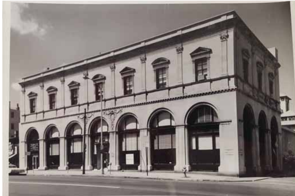
View from Massachusetts Ave
