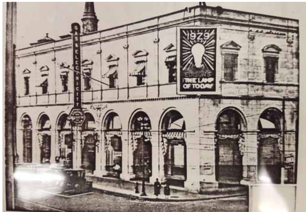
View from Massachusetts Ave
