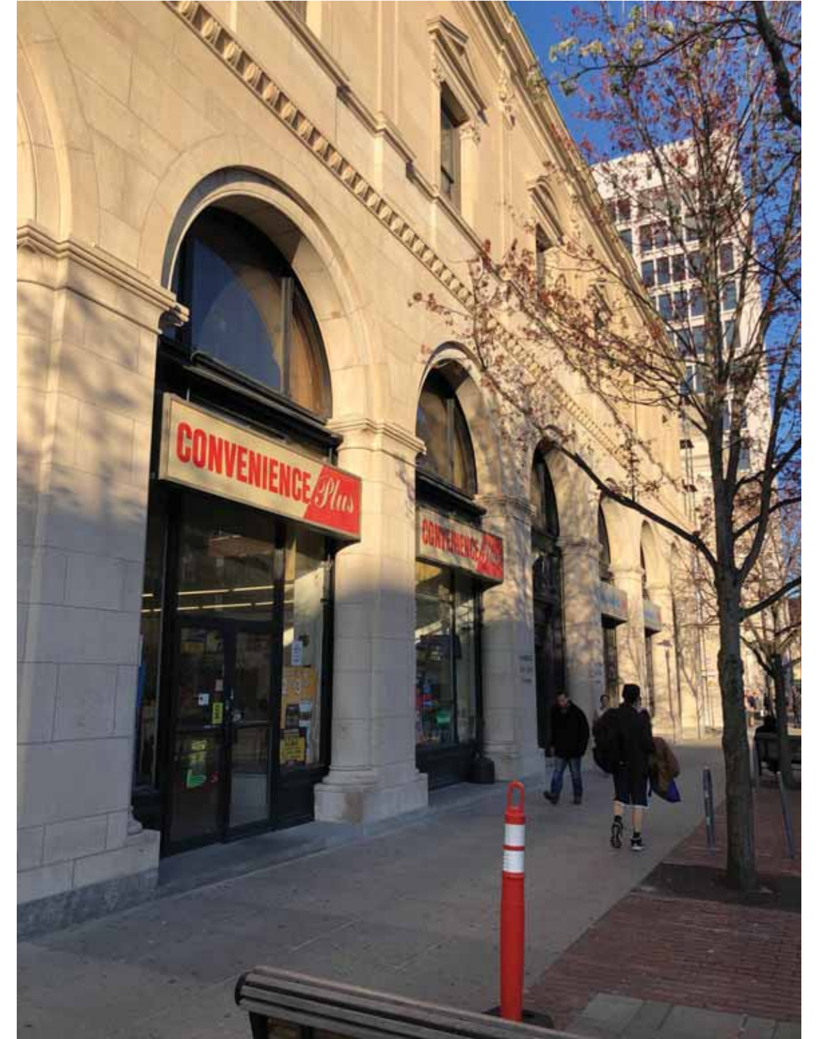
Closeup View from Massachusetts Ave Looking East
