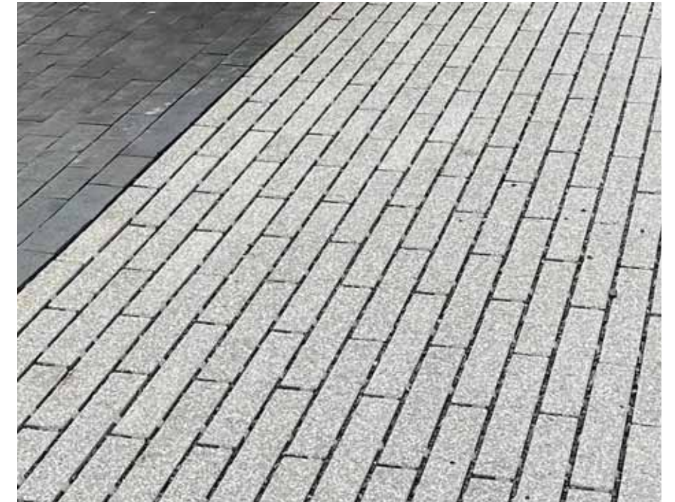
PERMEABLE UNIT PAVING
