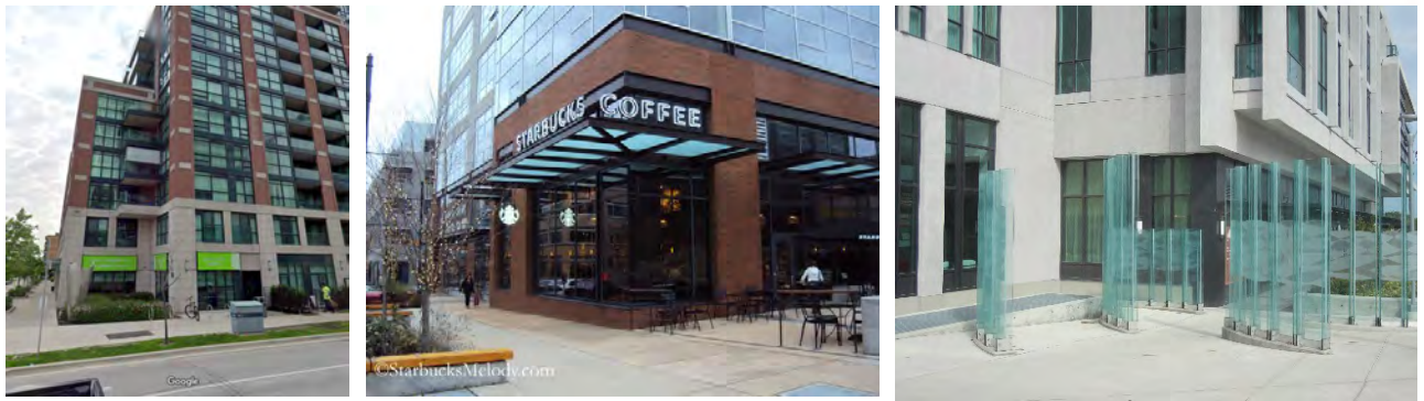
Image 7: Examples of Wind Control Measures at Building Corners
