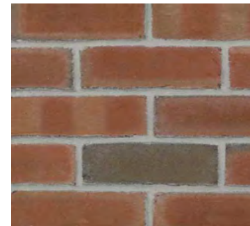
3 REBUILT BRICK WALL @ GREEN ST
