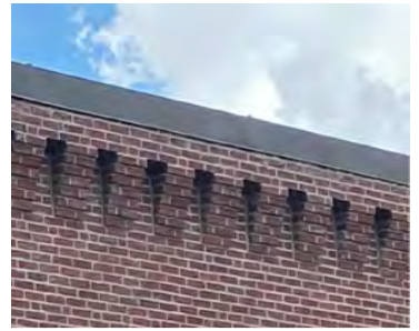
Photo of existing cornice to be replicated
