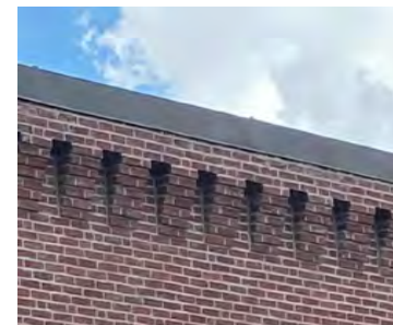
Photo of existing cornice to be replicated
