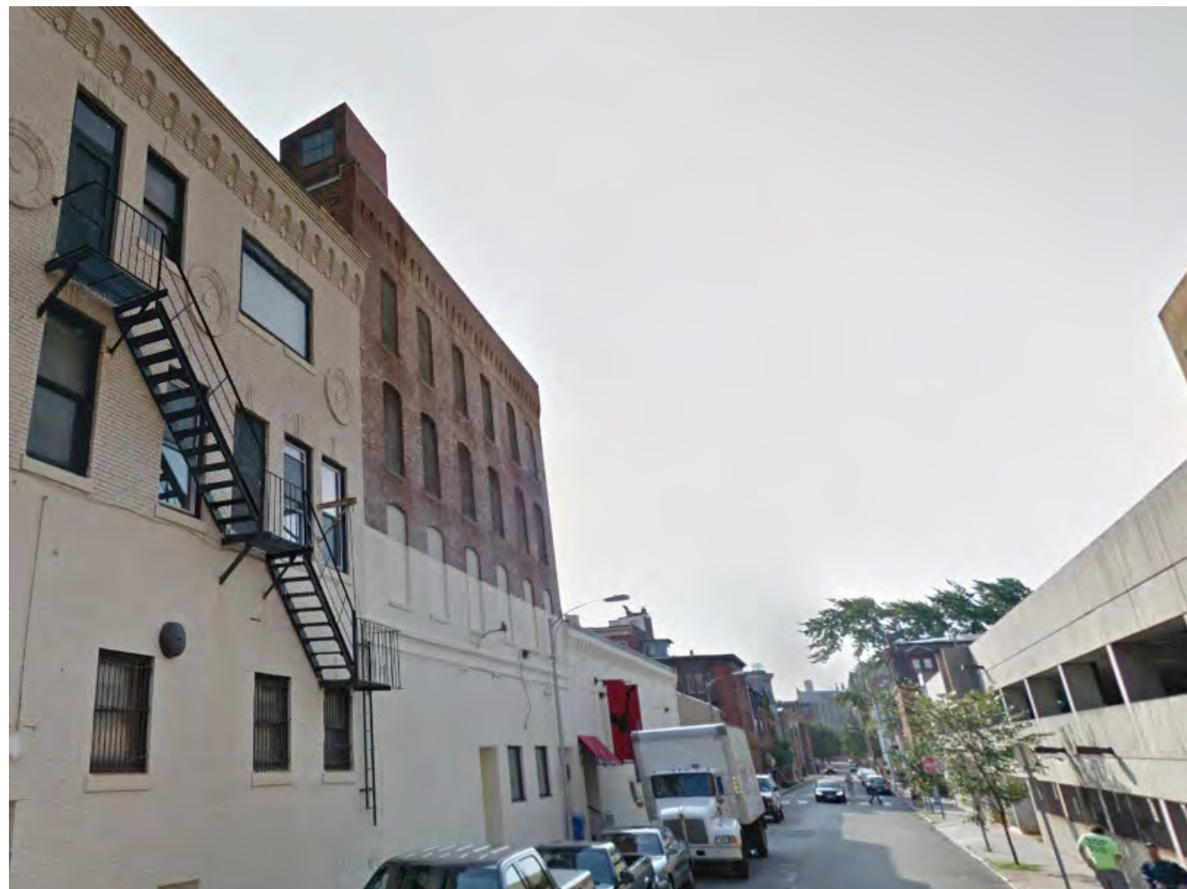
2. EXISTING GREEN ST. SOUTH WEST VIEW
