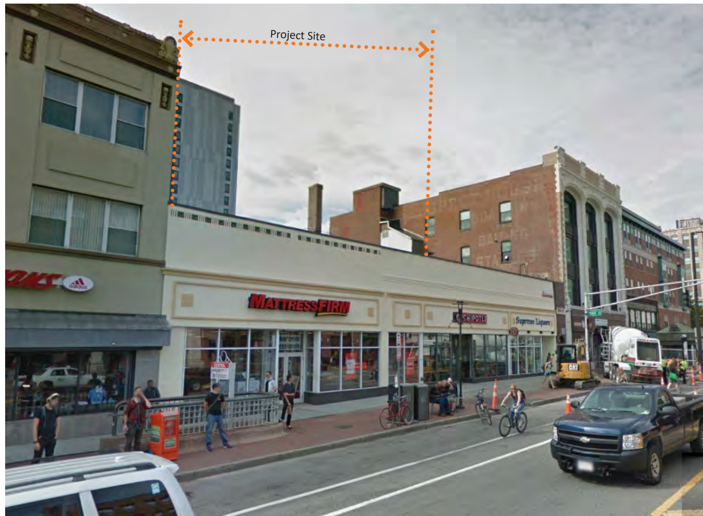
2. EXISTING MASS AVE. NORTH EAST VIEW
