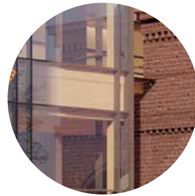
GLASS Curtain Wall
