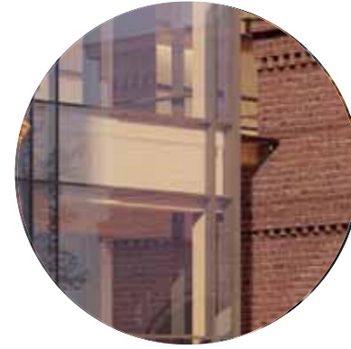
GLASS Curtain Wall
