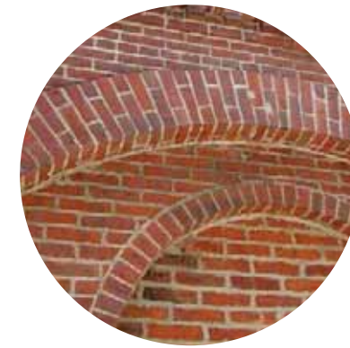
MASONRY Historic Brick
