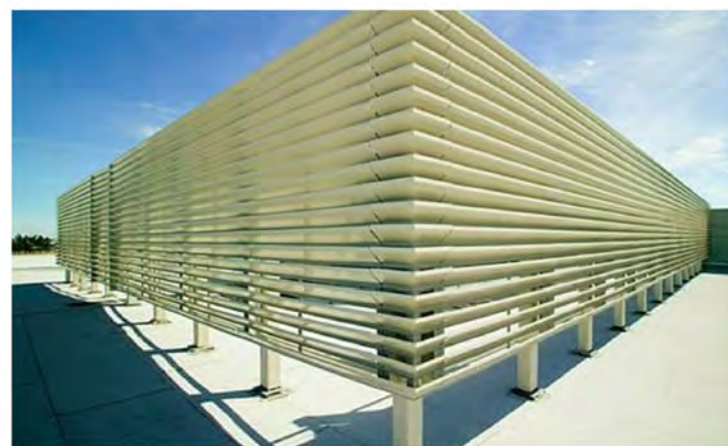
5. ROOFTOP ACOUSTICAL SCREENING
