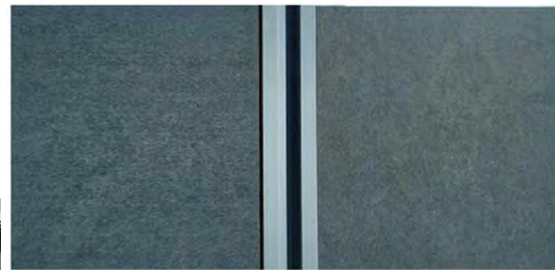
1. CEMENTICIOUS PANELS WITH REGLETS CEMBRIT (8mm) OR SIM; COLOR: FLINT USED AT BISHOP ALLEN/DOUGLASS CORNER PENTHOUSE LEVEL & ALL BALCONIES
