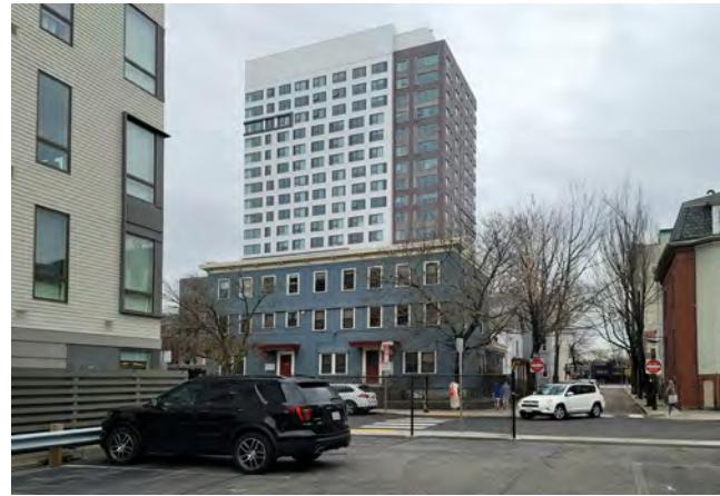
FRONT RIGHT SIDE OF BUILDING (BISHOP ALLEN DRIVE)
