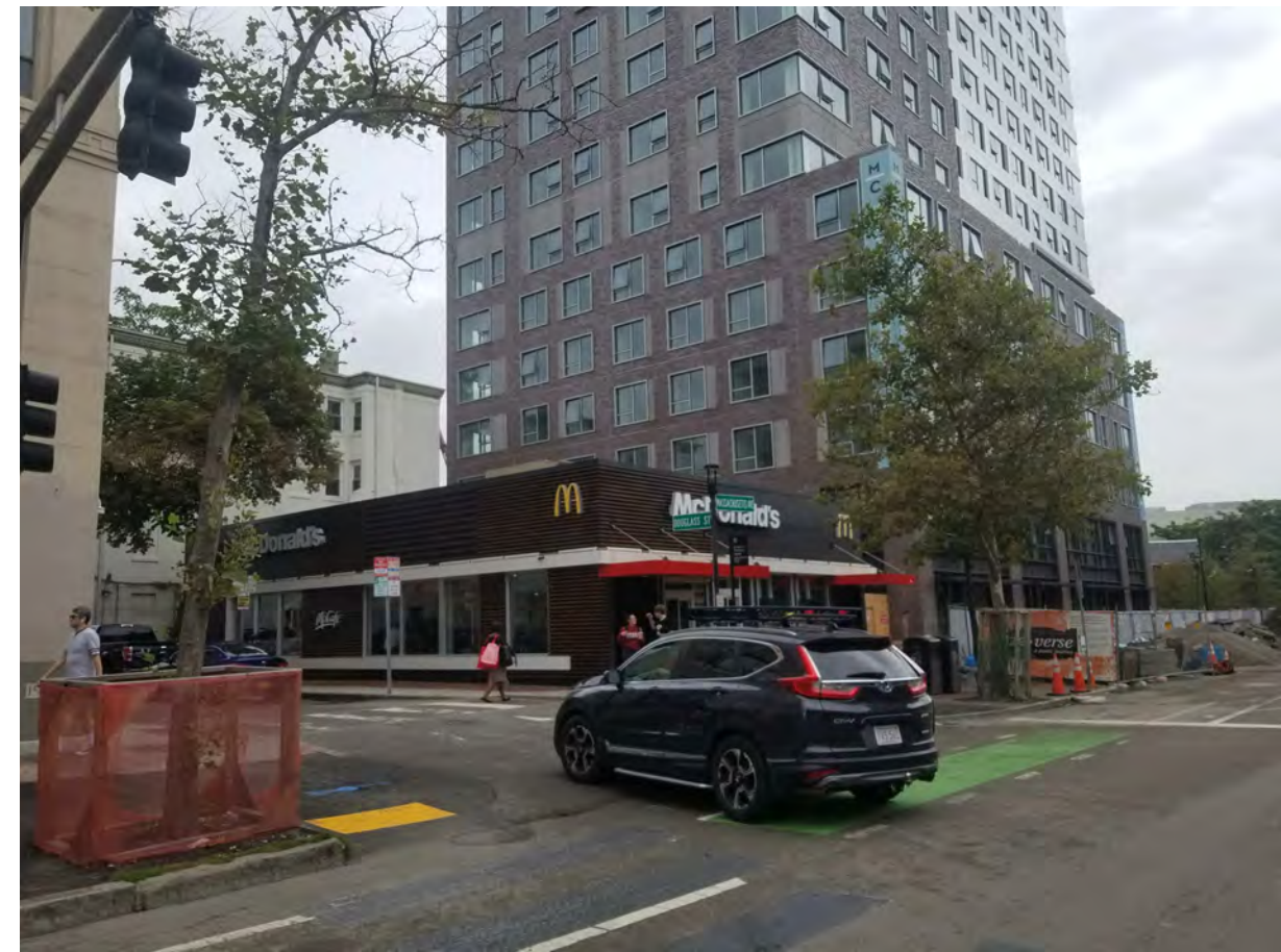
MARKET CENTRAL PROJECT FROM MASSACHUSETTS AVENUE AT BROOKLINE ST
