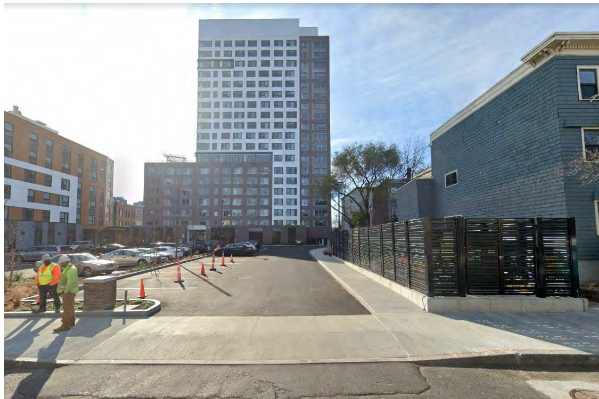
MARKET CENTRAL PROJECT FROM BISHOP ALLEN DRIVE
