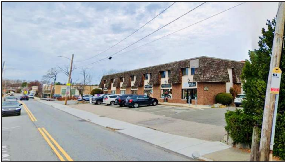
Photo of Existing Building Looking North
