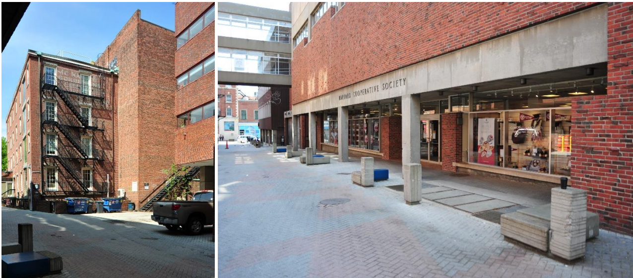
26 Church Street and the rear of the Harvard Square Theater (left); recessed storefronts of the Coop Annex (right)
