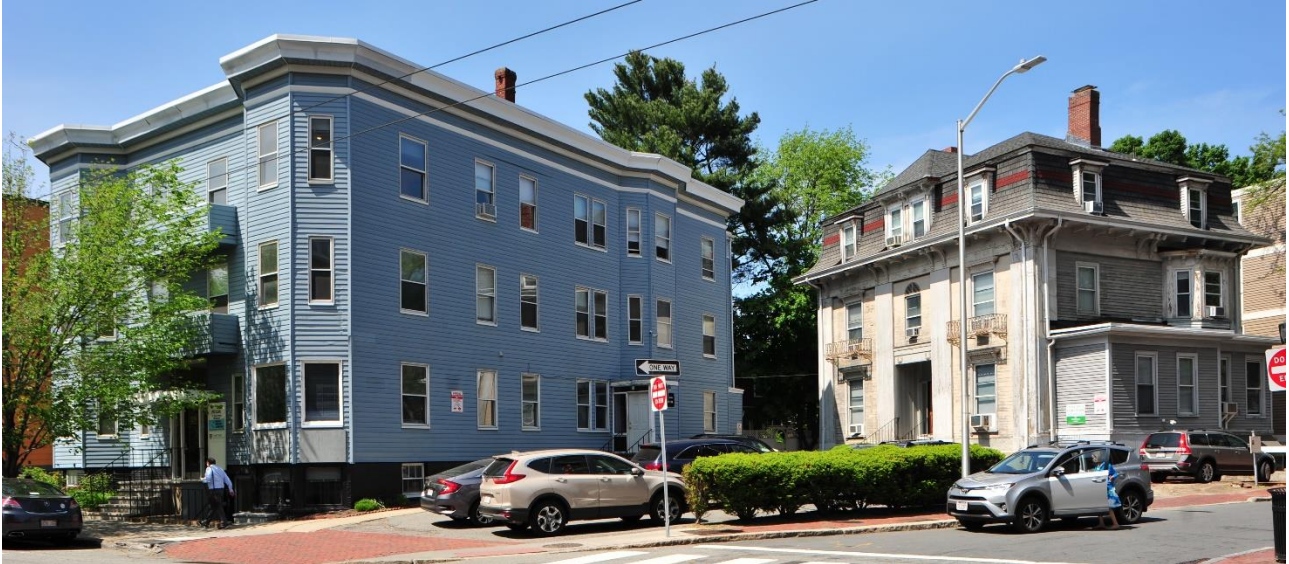
127 Mt. Auburn Street (1912) and the Munroe-Jacobs Jacobs house, 17 Story Street (1846).
