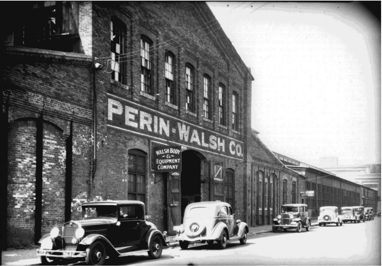
101 Rogers Street, Bent Street elevation, 1935
