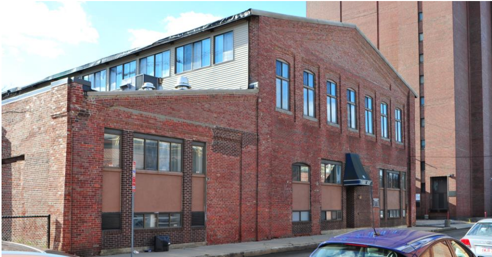
101 Rogers Street, north elevation
