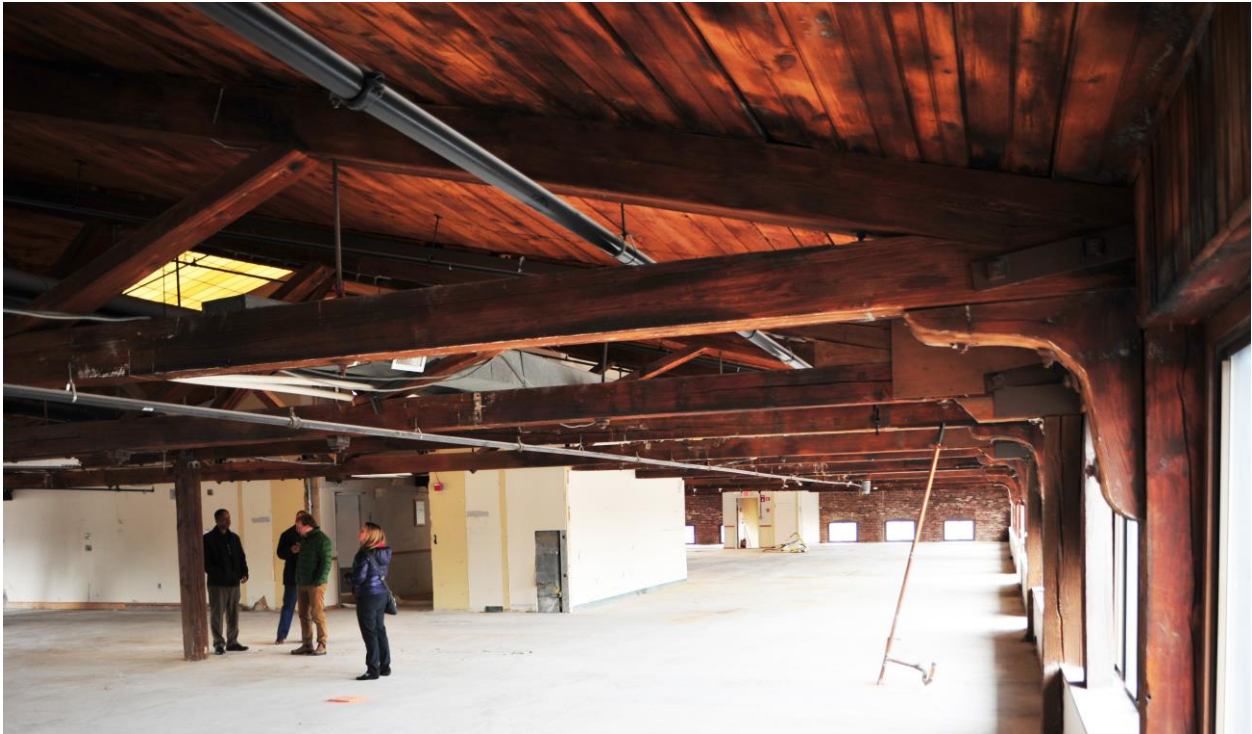
101 Rogers Street, second floor. Main roof framing.
