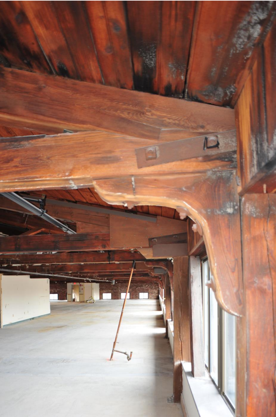
101 Rogers Street, second floor. Detail of roof framing.
