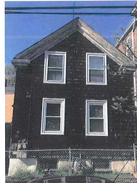
VIEW OF SOUTH (FRONT) ELEVATION
