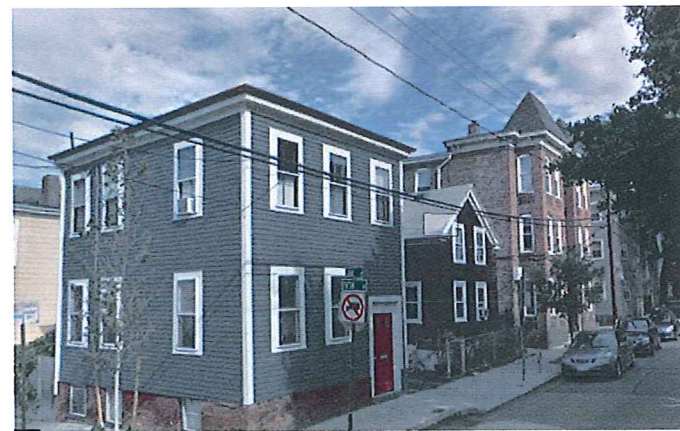
VIEW LOOKING EAST AT GORE ST. AND 5TH ST. INTERSECTION
