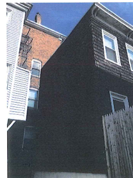
VIEW OF NORTH (REAR) ELEVATION
