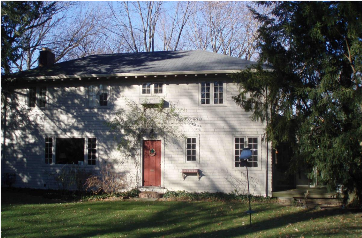
15 Gurney Street, Cambridge Assessor's Department East (front) elevation
