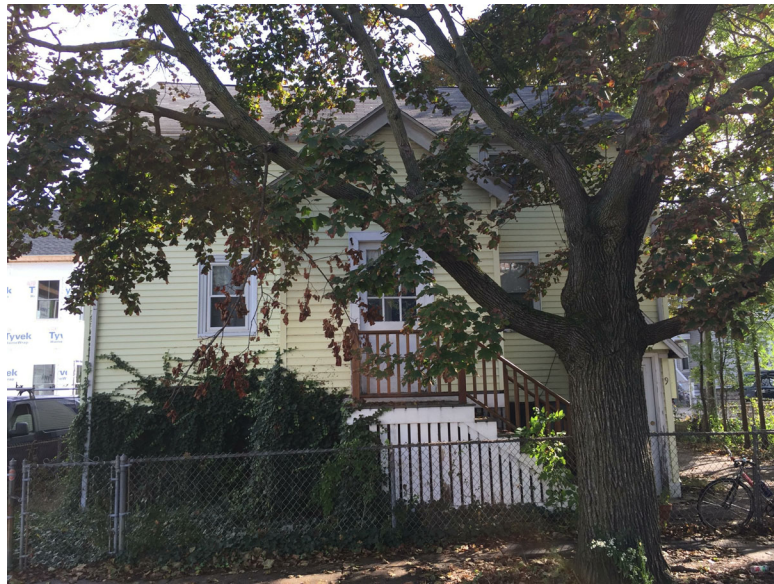
EXISTING JACKSON ST FACADE, WEST ELEVATION
