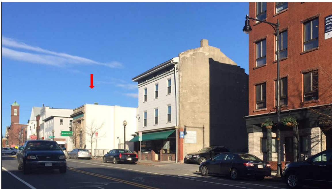
Cambridge St. looking west. 207 Cambridge St. (Gould House and Bakery of 1857) at center and 227 Cambridge St. (Lechmere National Bank) marked with arrow at left.
