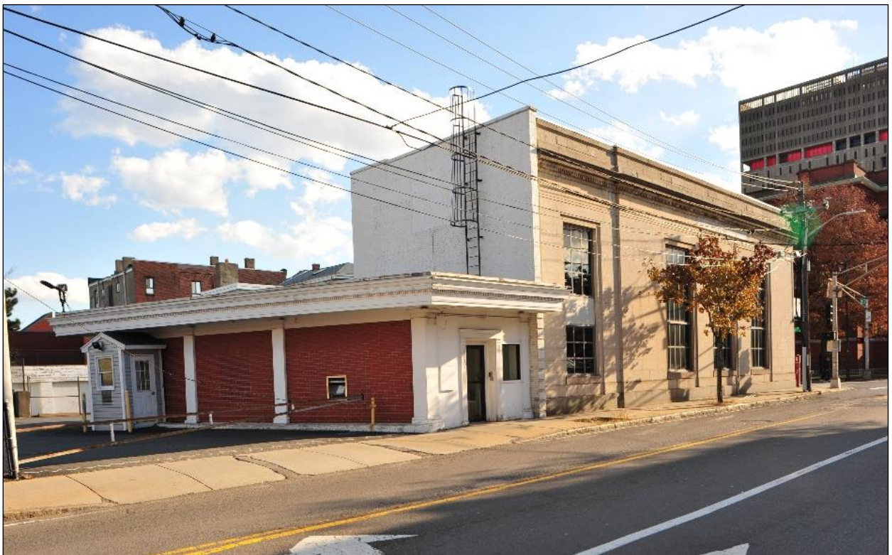
North (rear) elevation, November 2017. Rear addition (1961) is to be removed.
