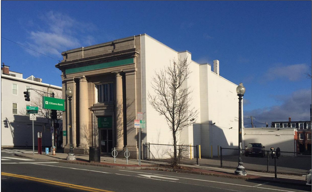
South (front) and east elevations, February 2017.
