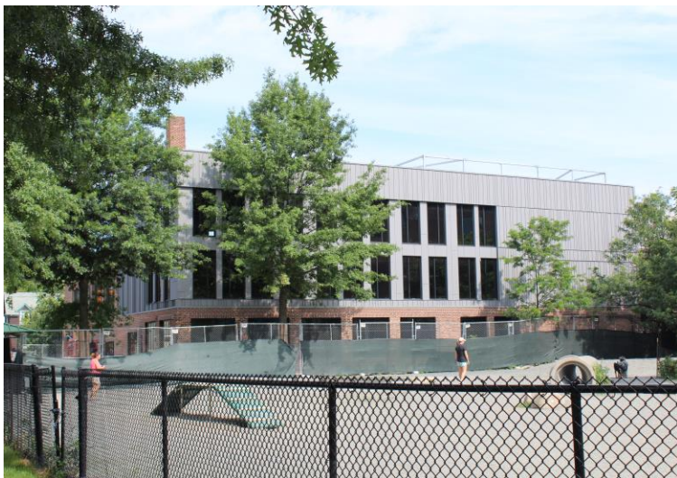
Previously approved cladding and new sash. Tudor Street façade (top) and viewed from Tudor Street Dog Park (bottom). CHC staff photos, August 1, 2019.
