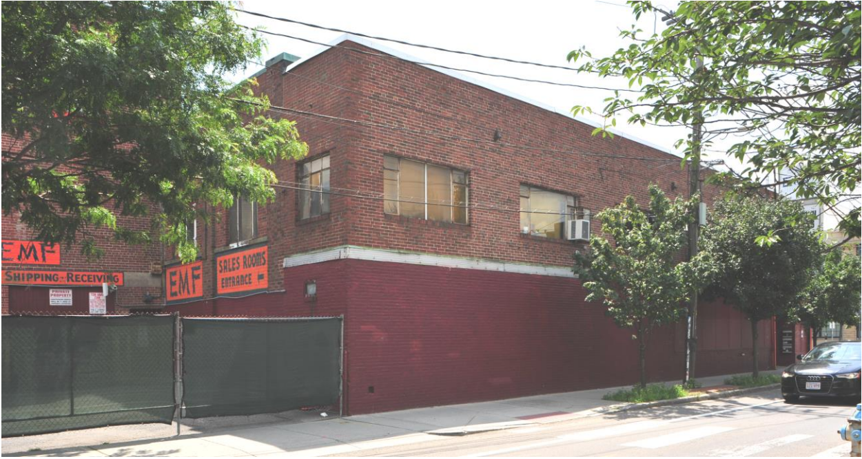
EMF Building, 116 Brookline Street, July 2018.
