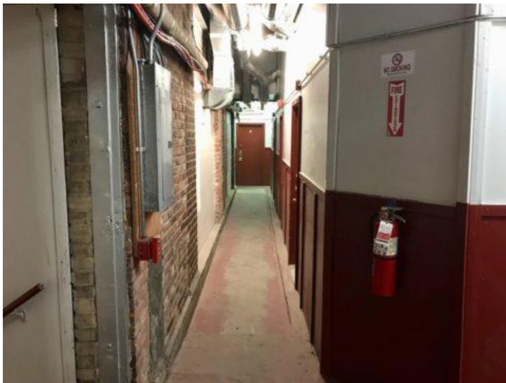
116 Brookline Street, interior corridors constructed for musicians' studios. Cambridge Day , April 28, 2018
