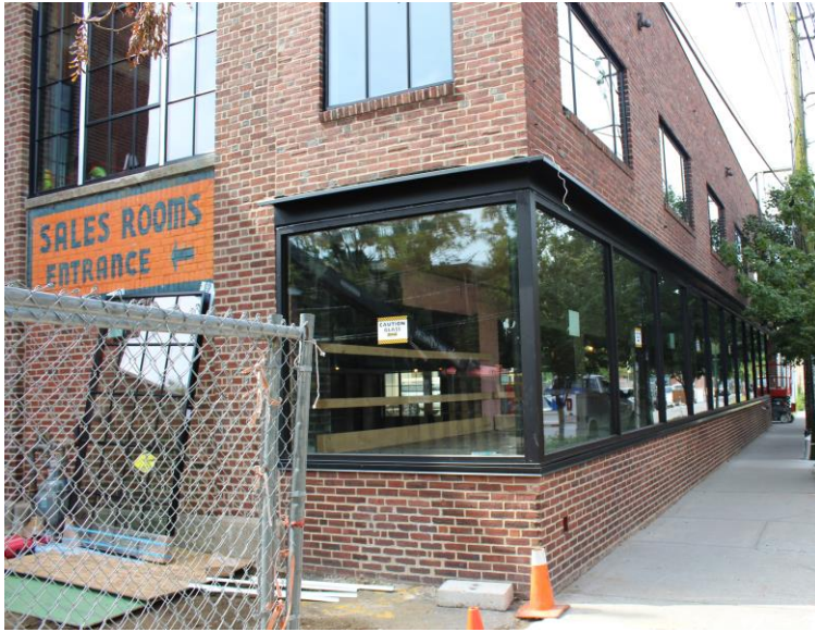
Existing painted signs and previously approved replacement storefronts.
