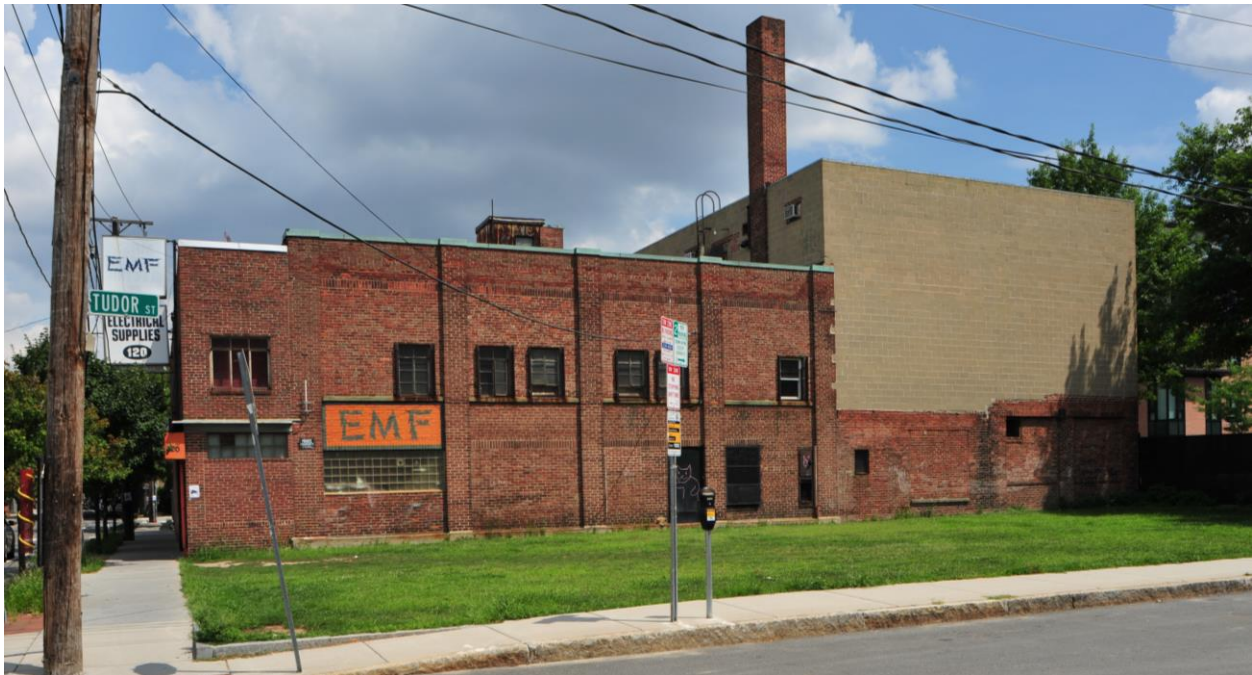
EMF Building, 116 Brookline Street, July 2018
