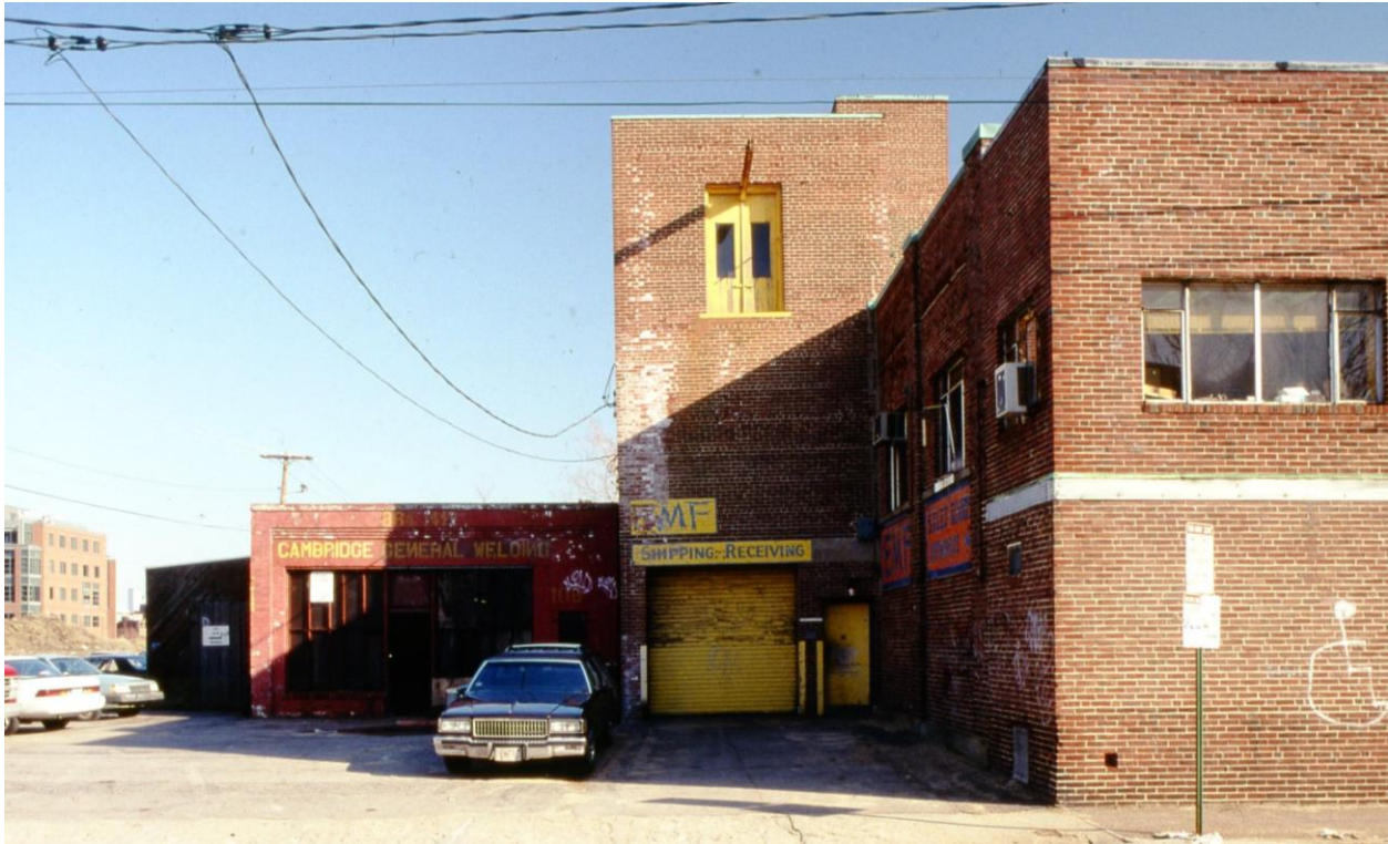
116 Brookline (right) and 112 Pacific Street (left) in 1994 photograph. Note the enclosed bricked-up storefronts at right.
