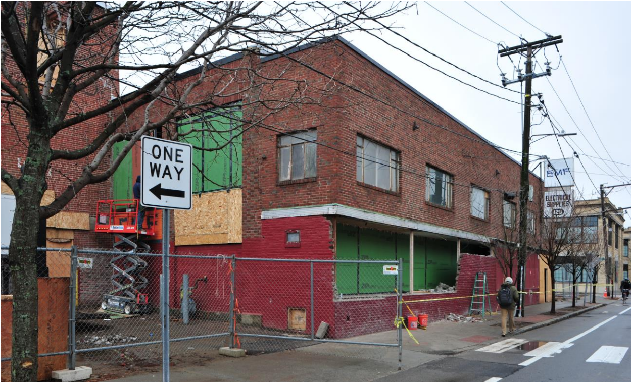
EMF Building, 116 Brookline Street, February 2019
