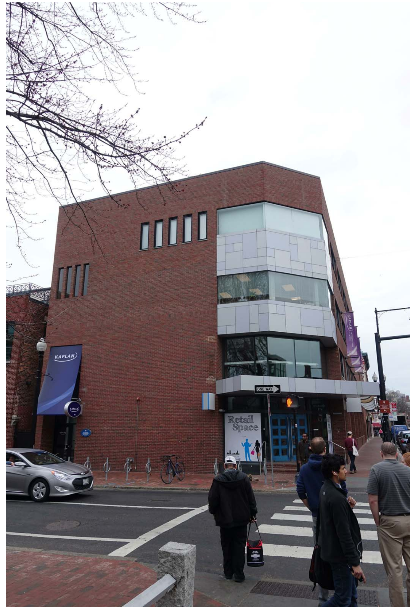
EXISTING EXTERIOR PHOTOGRAPH
