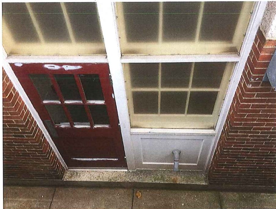
Areaway Entry to Schlesinger Basement
