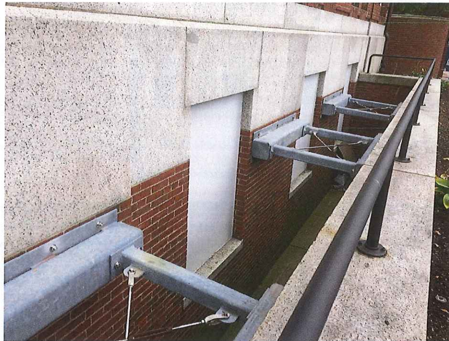
Looking South into Areaway
