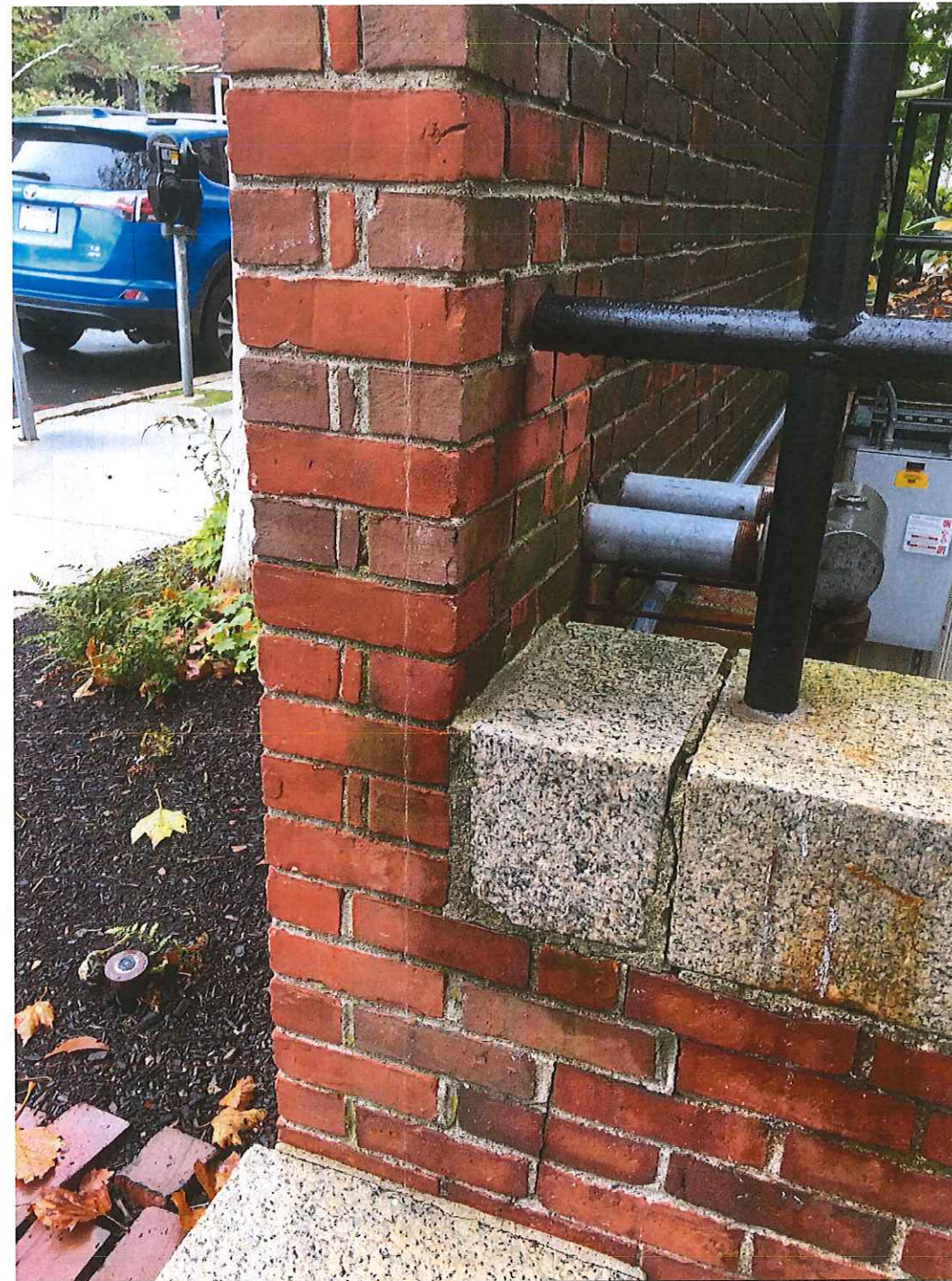
Existing Extended Wall at North End of Areaway
