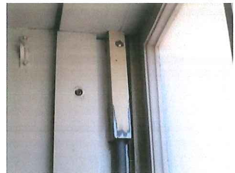
Group B- Lower sash tube spring balance
