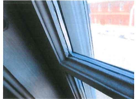
Group A- Retrofitted insulated glass
