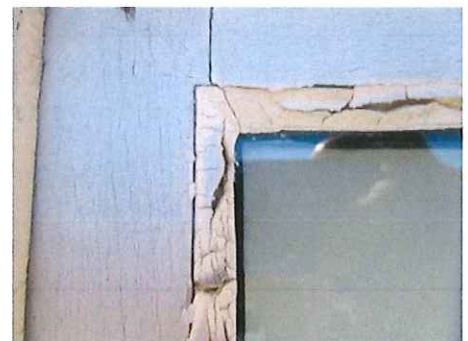
Group A & B- Sash cut for IGU
