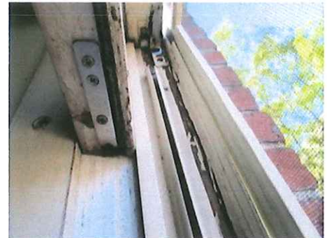
Group B- Upper sash plastic spring balance jamb, and lower sash tube spring balance with aluminum jamb
