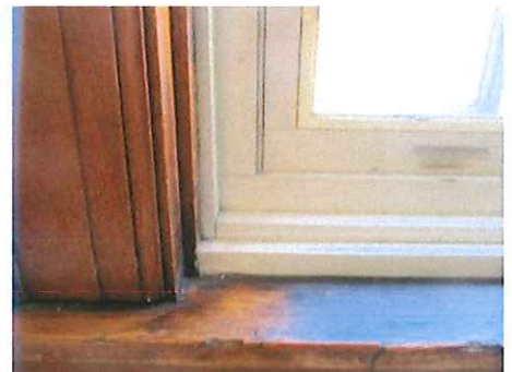
Group C- New window insert's jamb and balance extends past the original jamb by about 1”
