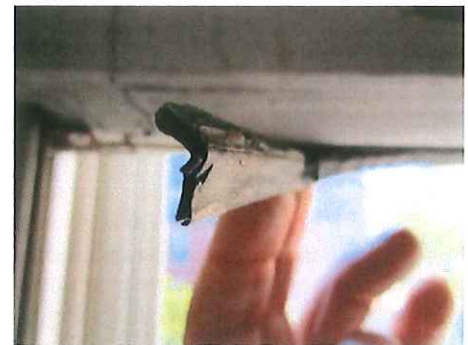
Group A & B- Bottom sash weather stripping
