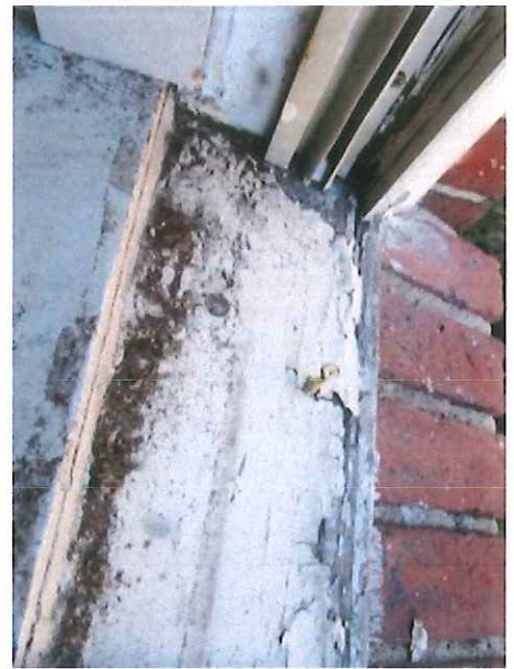
Group A, B, & C- Sill require scraping, consolidation, and refinishing
