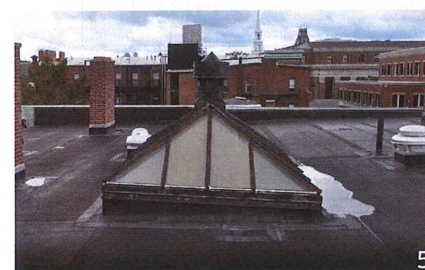
EXISTING SKYLIGHTS AND BULKHEAD
