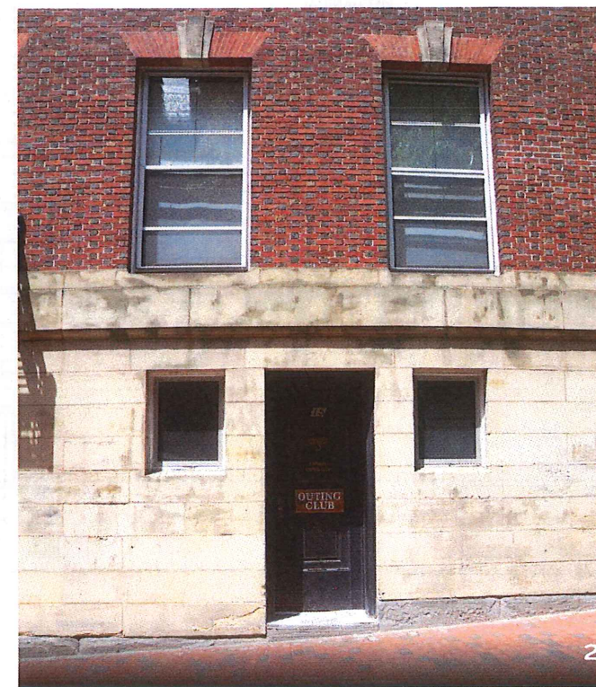
EXISTING OUTING CLUB DOOR
