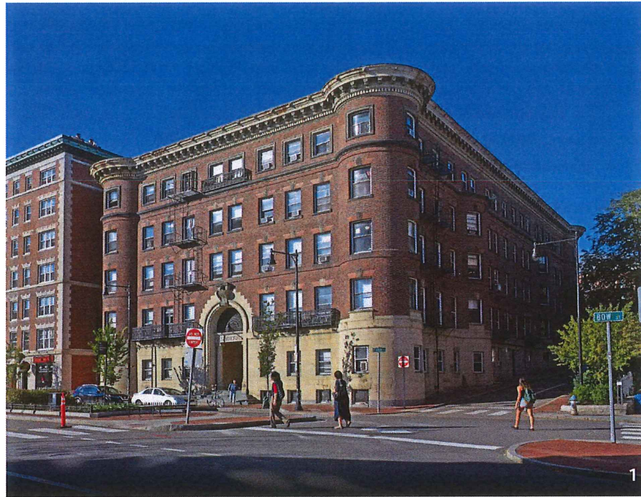
AT MT AUBURN/BOW STREETS - LOOKING NORTHWEST
