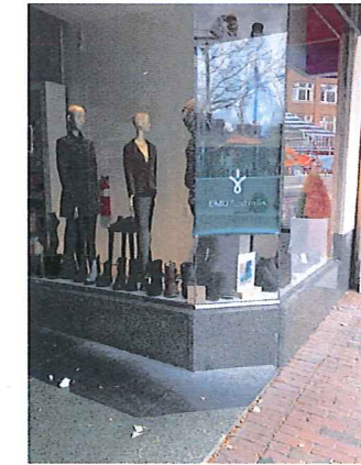
29 BRATTLE STREET, CAMBRIDGE, MA 02138 2019. 11.18 EXISTING STONE BASE TO REMAIN AND TO BE CLADDED WITH BLACK METAL.
