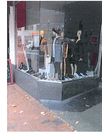
29 BRATTLE STREET, CAMBRIDGE, MA 02138 2019. 11.18 EXISTING STONE BASE TO REMAIN AND TO BE CLADDED WITH BLACK METAL.
