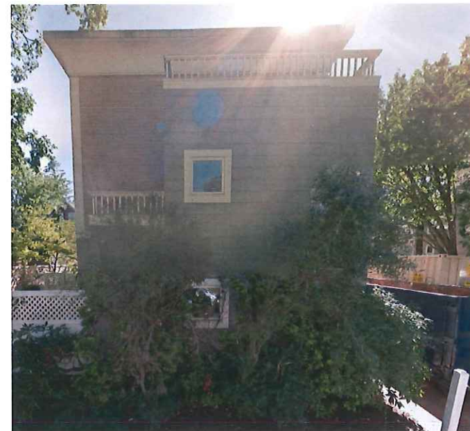
243-245 CONCORD AVE. (seen from RC Kelley)
