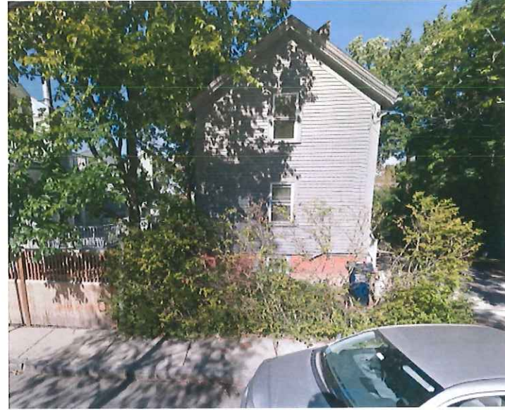
7 R.C. KELLEY STREET (existing)
