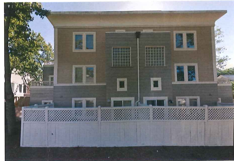
243-245 CONCORD AVE. (seen from RC Kelley)
