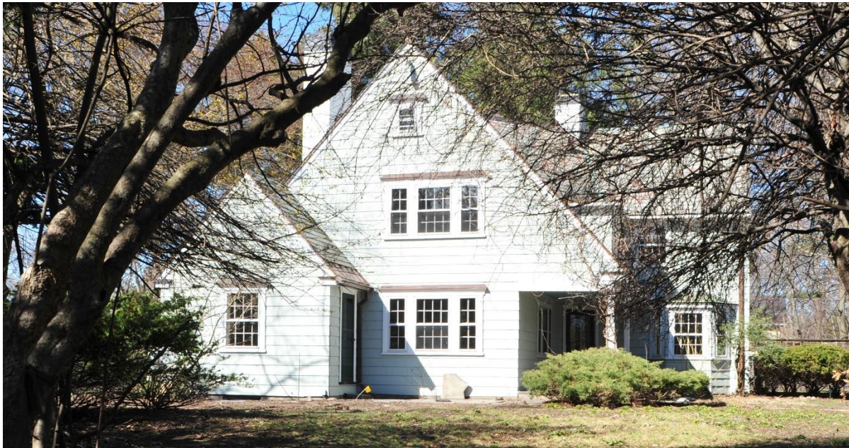
127 Coolidge Hill, south elevation
