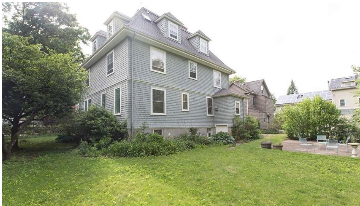
247 Lakeview Avenue, rear yard and southeast corner MLS # 72016621 listing photo from Estately.com
