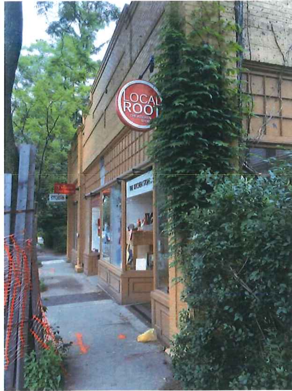
221-225 CONCORD AVE EXISTING RETAIL
