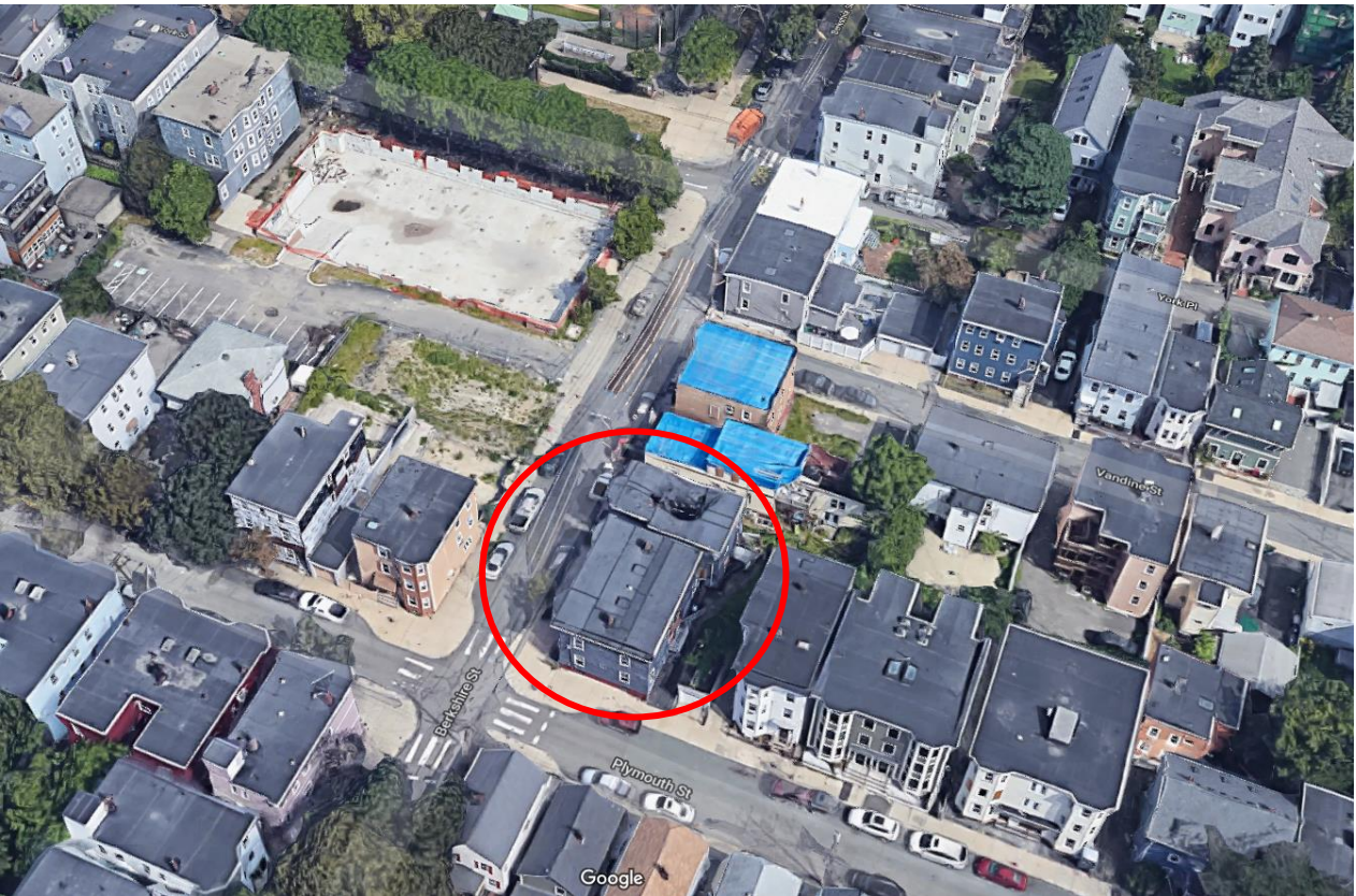
Berkshire Street neighborhood post-fire
