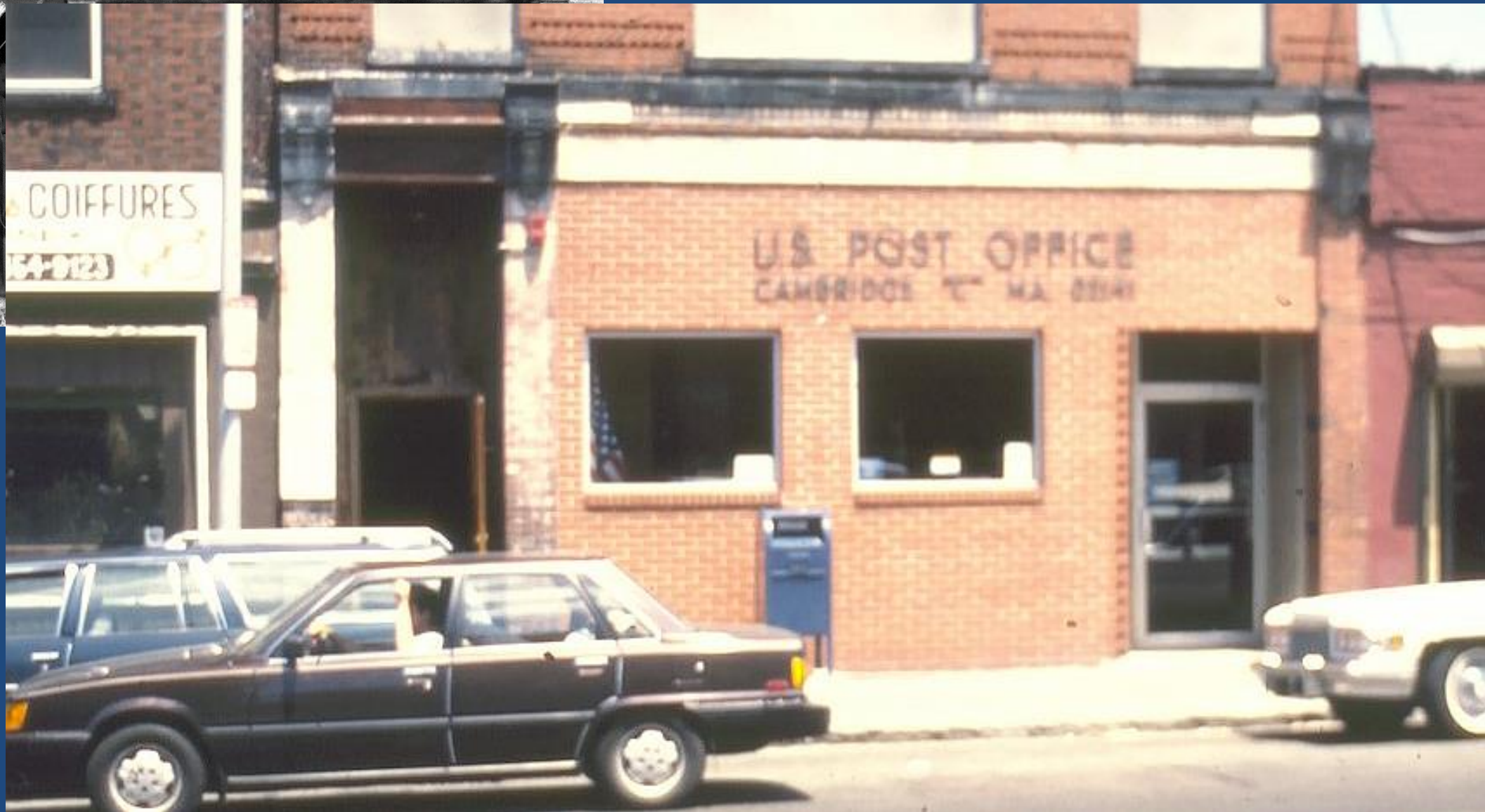
305 Cambridge Street. Storefront 1975; photo 1983
