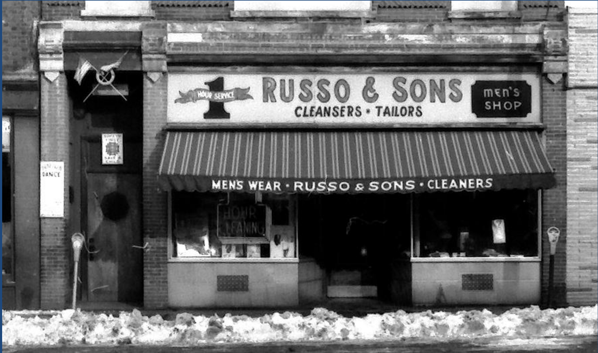
305 Cambridge Street. Storefront 1951; photo 1964
