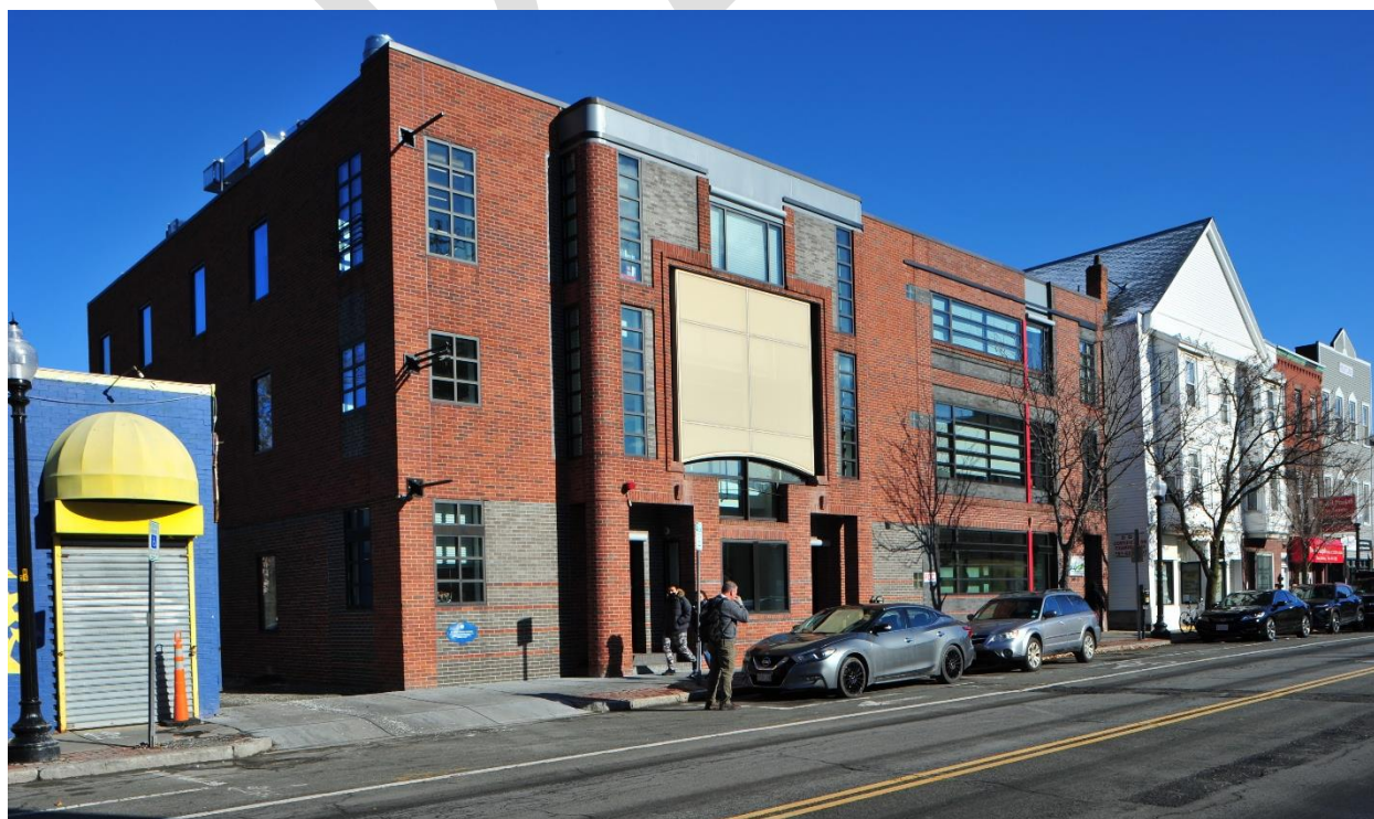
Case 4323: 271 Cambridge Street after renovation.
