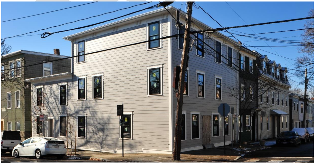
Case 4267: 118 Spring Street after renovation.
