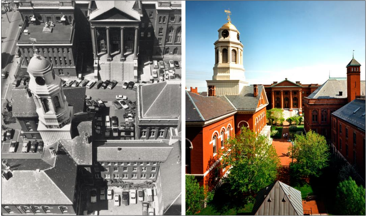
Middlesex County Complex – Bulfinch Square before and after 1984 restoration by Graham Gund.
