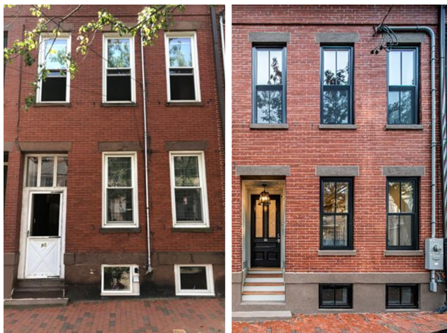
90 Thorndike Street façade before and after permit review.
