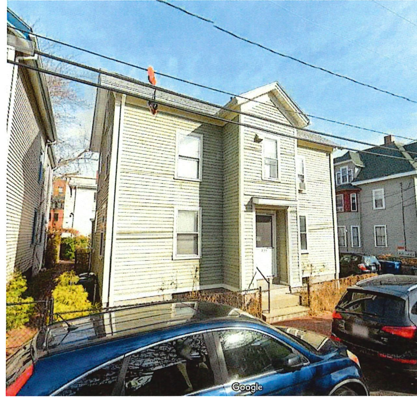
EXISTING STRUCTURE VIEWED FROM STREET
