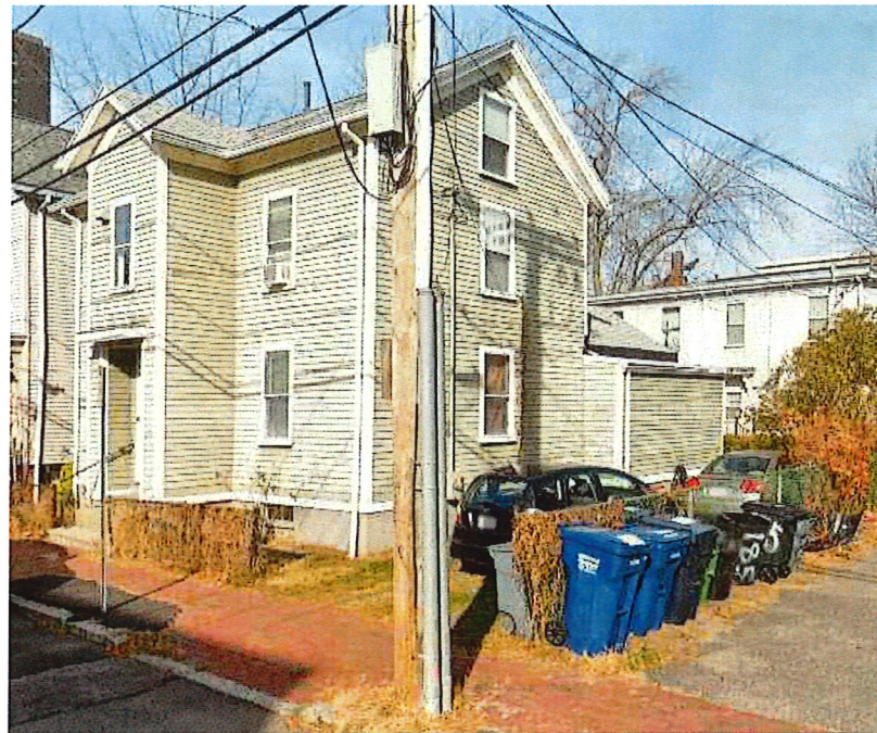
EXISTING STRUCTURE VIEWED FROM STREET
