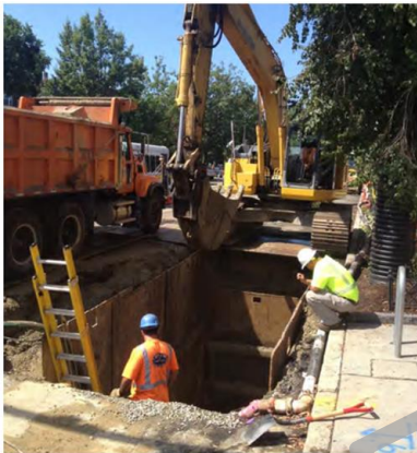
Trenching along Beacon Street, Brookline, August 2012
