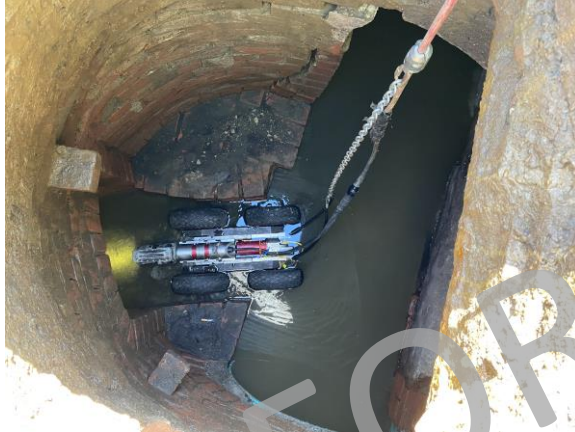
Pipe Inspection Equipment Entering Pipe to Assess Condition & Identify I/I
