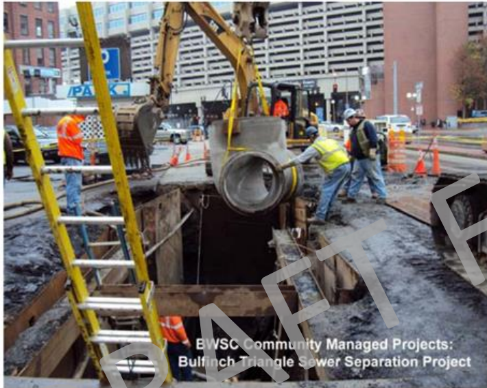
Installation of storm drain on Merrimac Street
