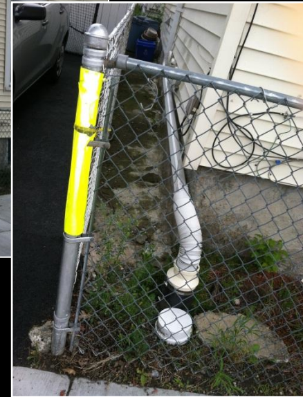
After: Downspout reconnected to new drain lateral with cleanout access. Sidewalk, driveway restored.
