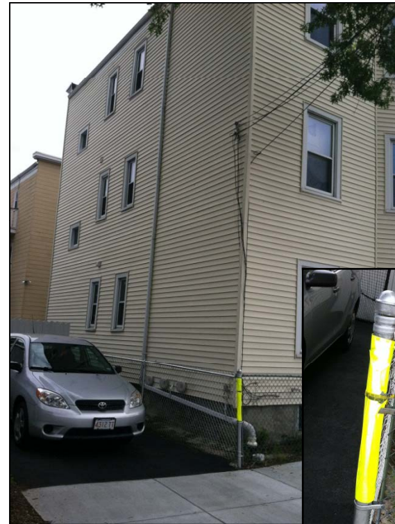
After: Downspout reconnected to new drain lateral with cleanout access. Sidewalk, driveway restored.
