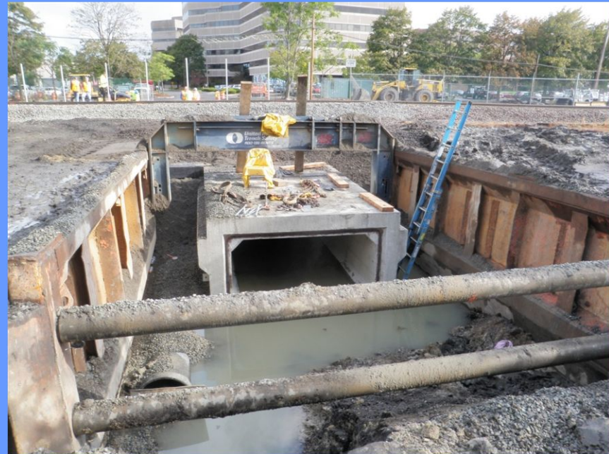
Box culvert installation at railroad crossing
