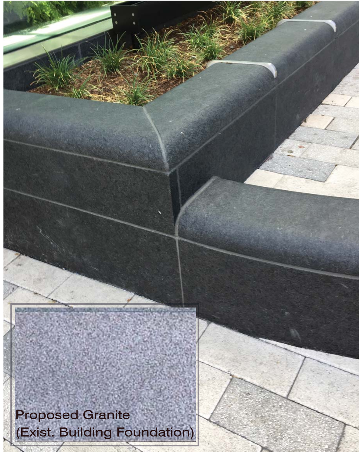
Eased/Radial Cheek Wall Edge Condition
