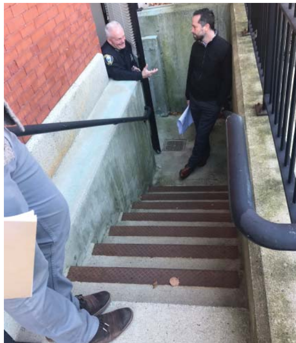
Existing Stair - To Remain
