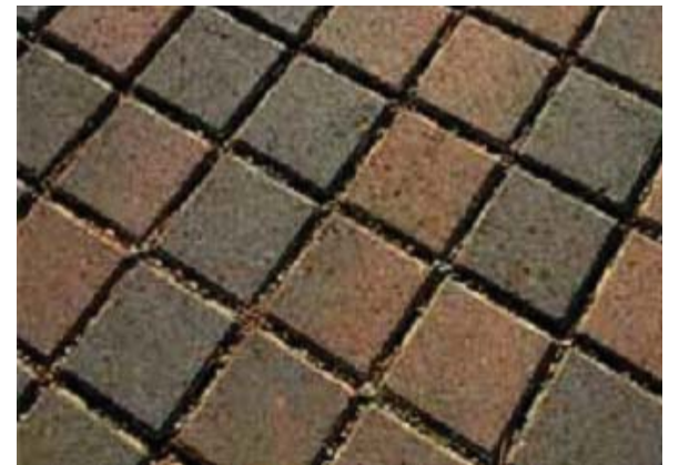
Permeable Conc Paver (Sand-based Structural Soil)
