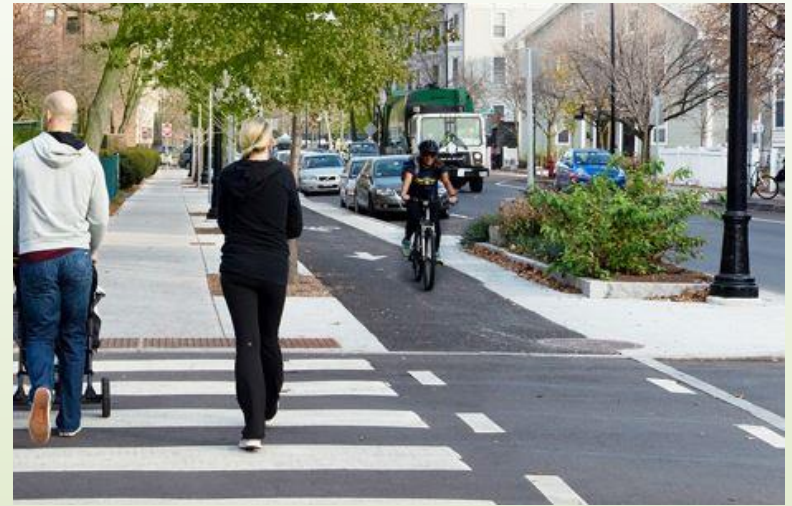
Protected Bike Lane
