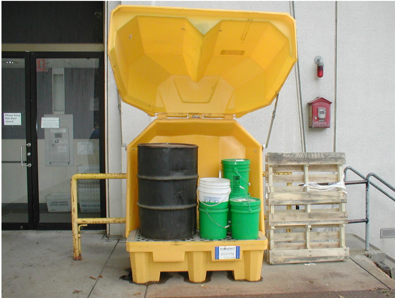
Example of shelter to protect oil containers
