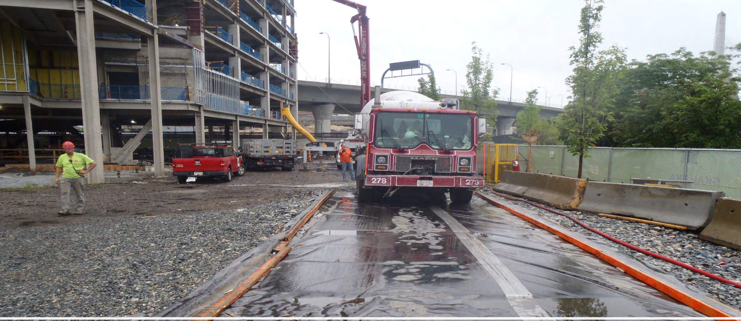
Construction Site entrance/exit crushed Stone
