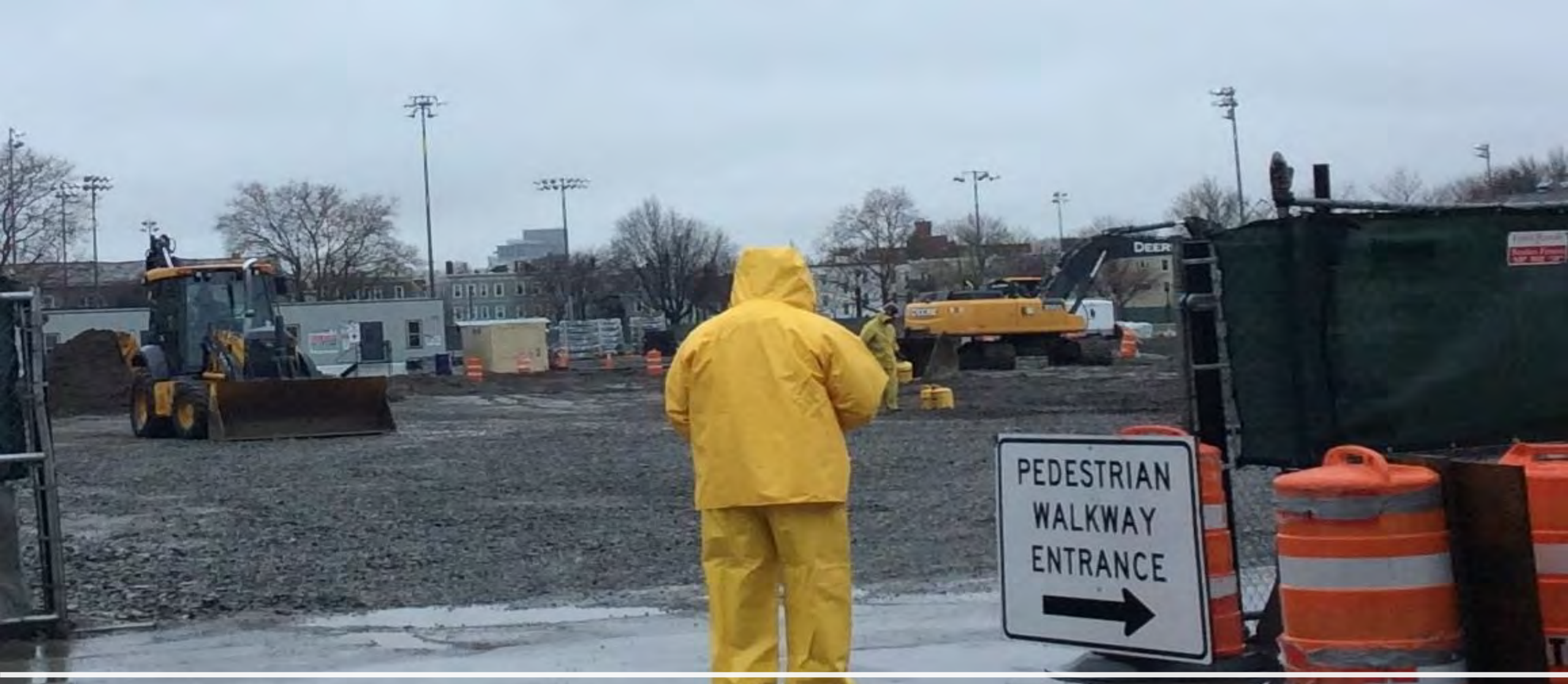
Construction Site entrance/exit crushed Stone
