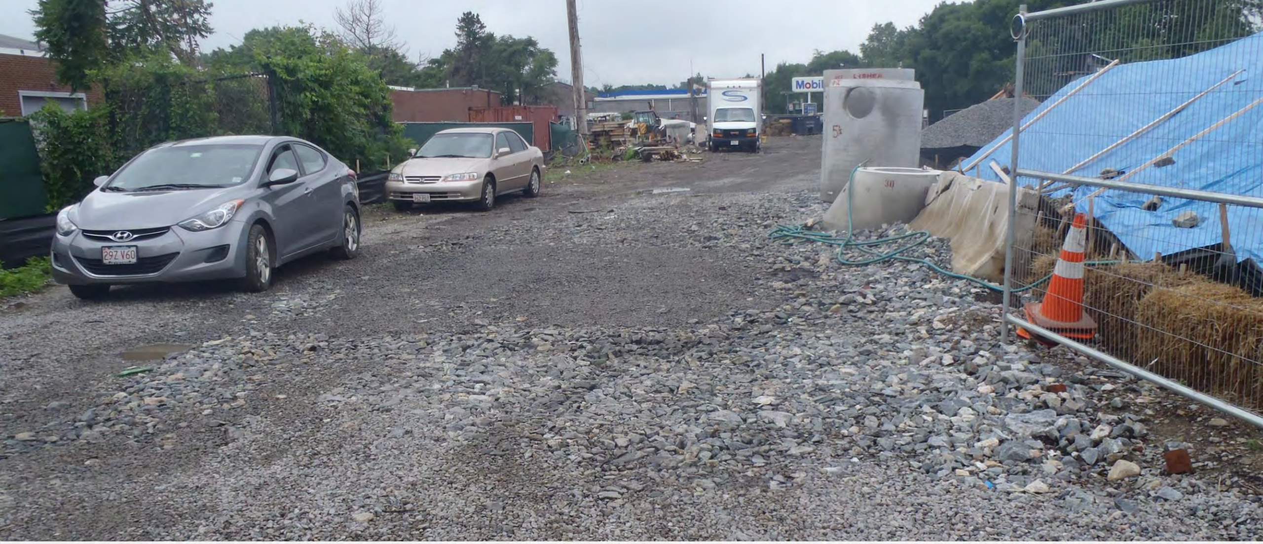
Construction Site entrance/exit crushed Stone
